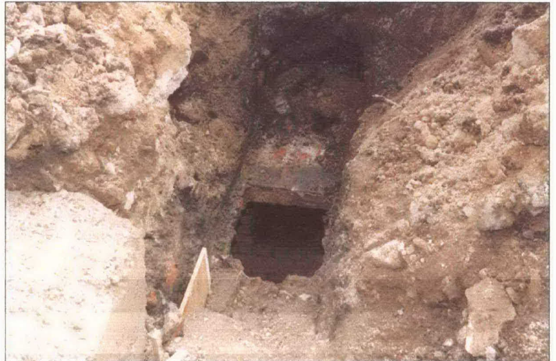
Plate 2 Top of exposed vaulted roof
