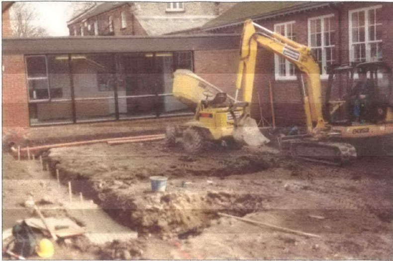
Plate 1 Looking south-east across excavations
