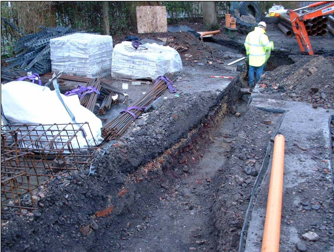
Plate 5. Trench 3 drainage trench looking southeast.
