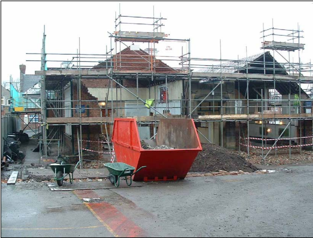
Plate 1. Trench 1, footprint of school building extension looking north.
