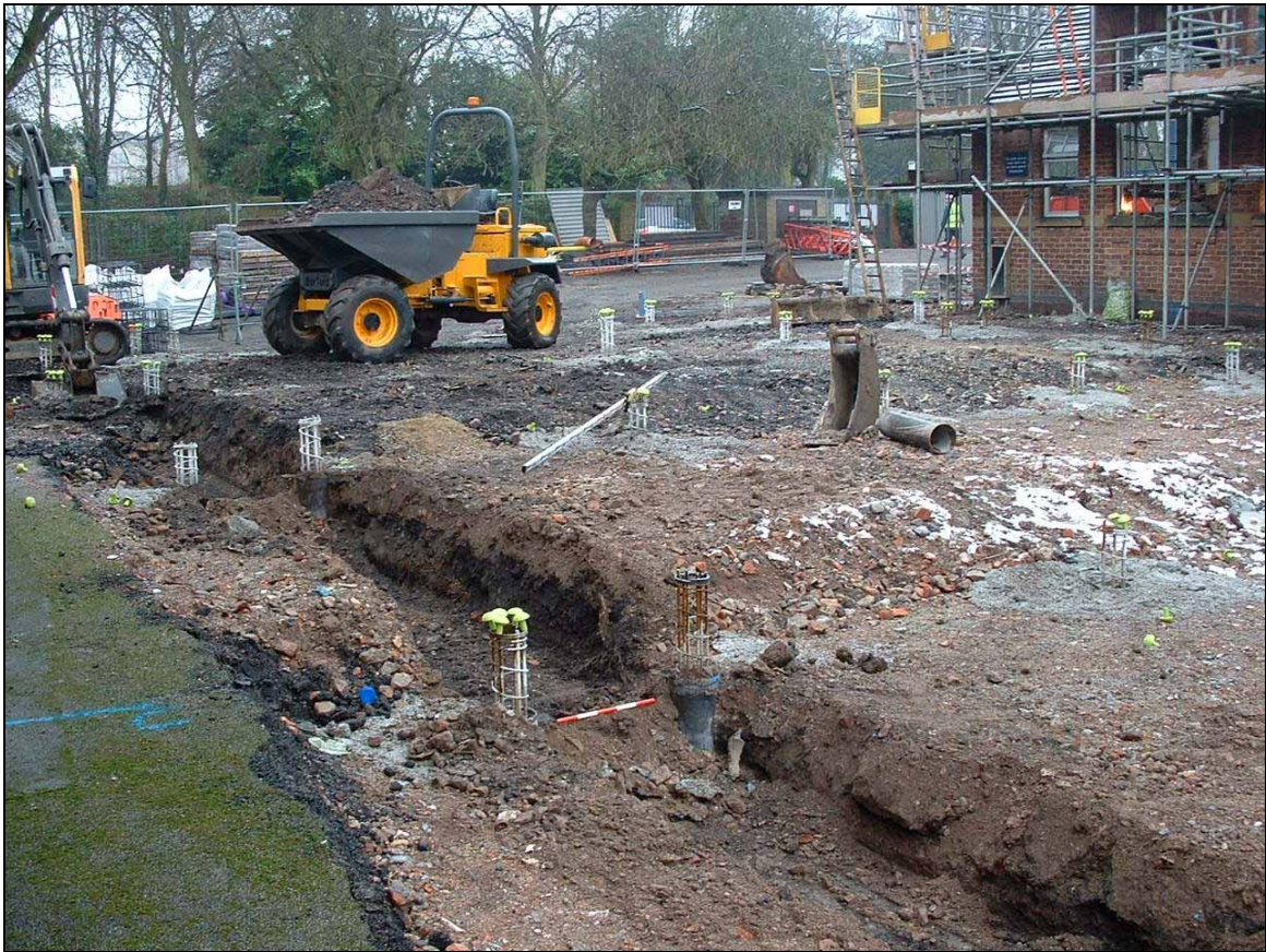
Plate 3. Trench 2 linking trenches looking southwest.
