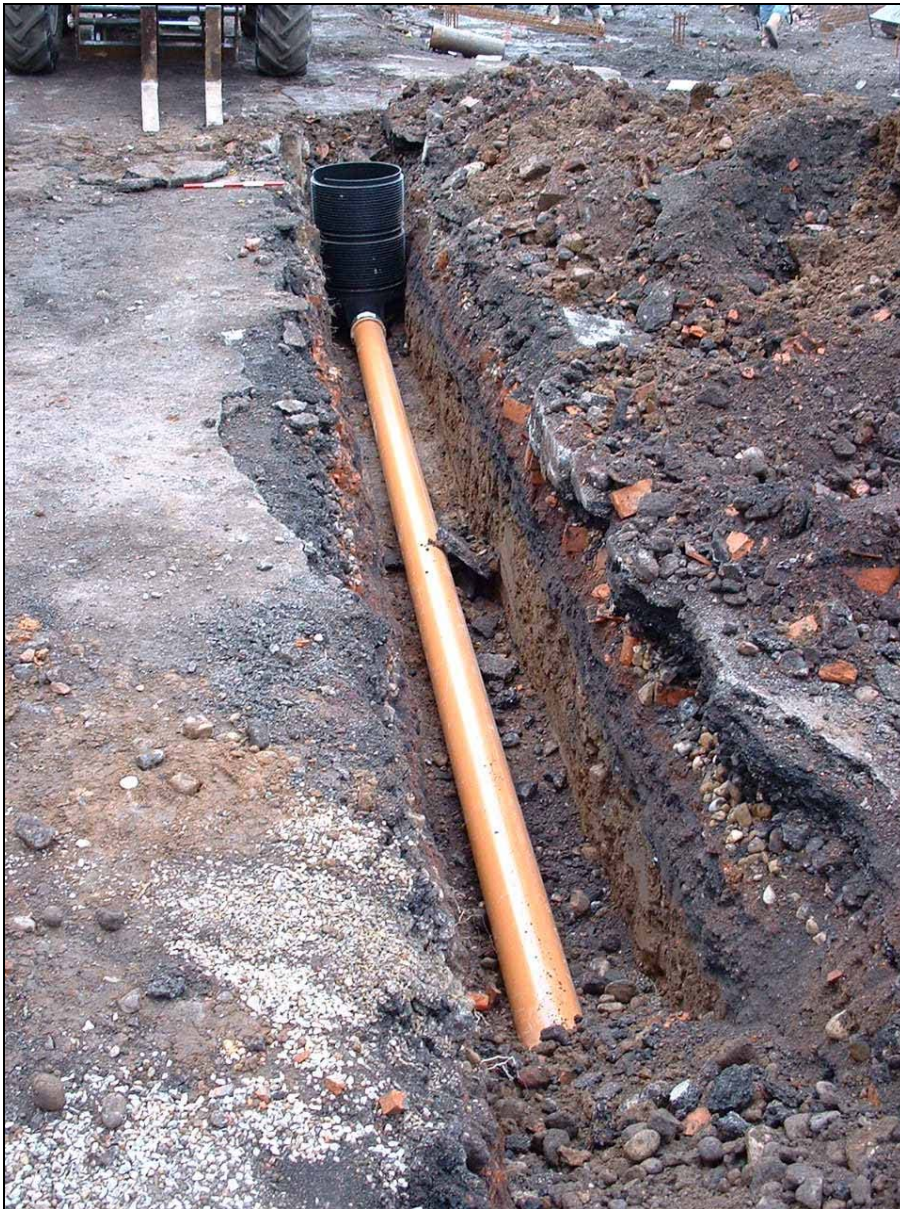
Plate 7. Trench 4 drainage trench looking west.
