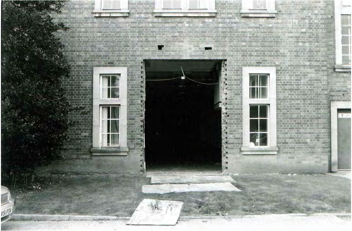
Plate 131. Factory. East Elevation. Facing West.
