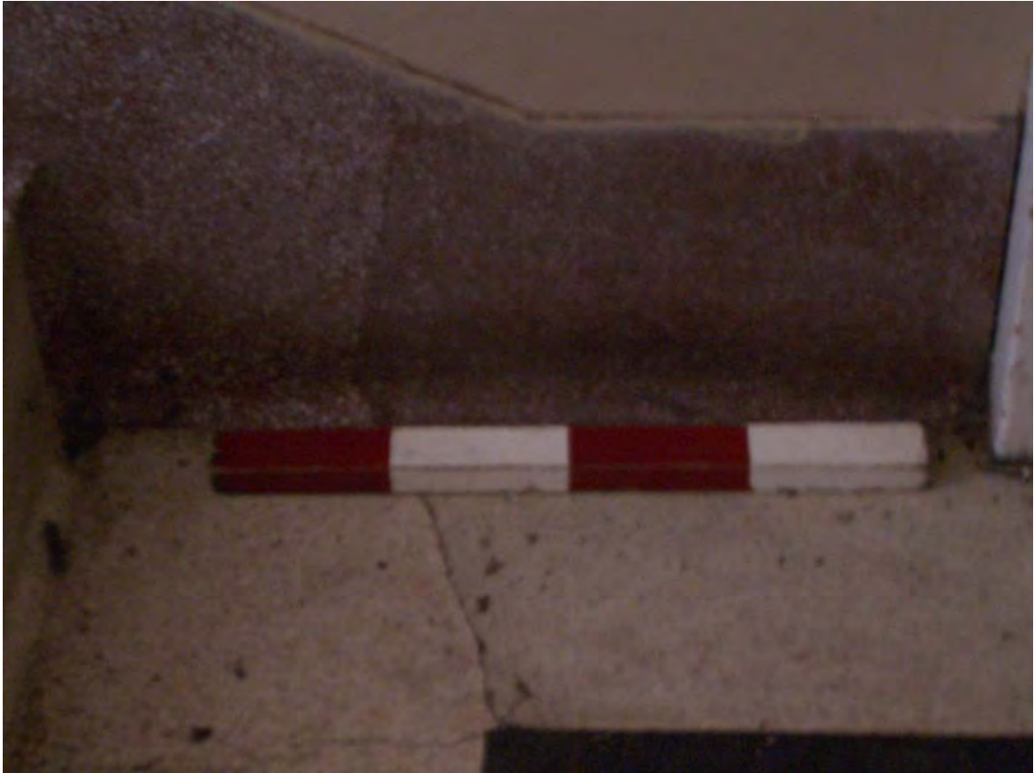
Plate 69. Head Office. First Floor Interior. Facing North.
