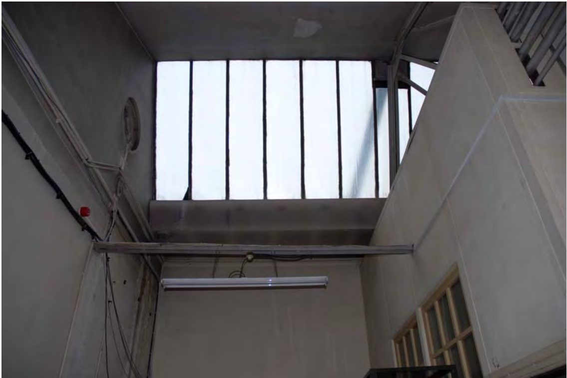
Plate 114. Head Office. First Floor Interior. Facing North.
