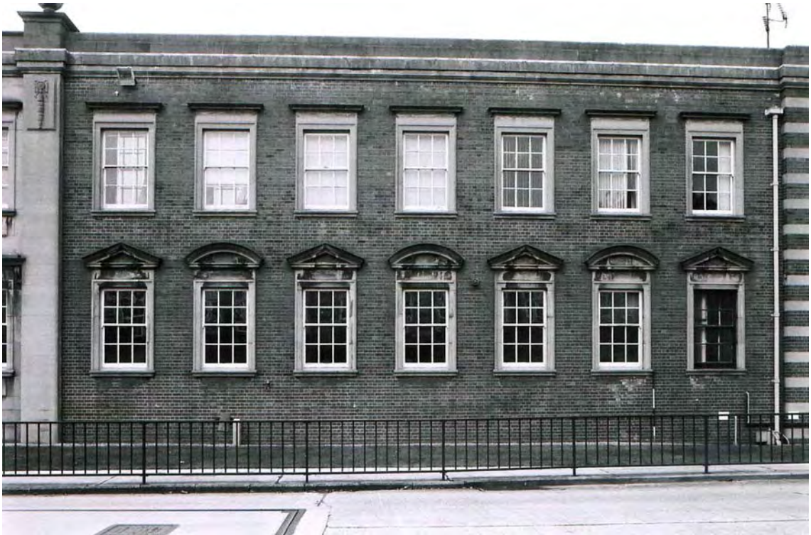
Plate 21. Head Office. South Elevation Windows. Facing North.
