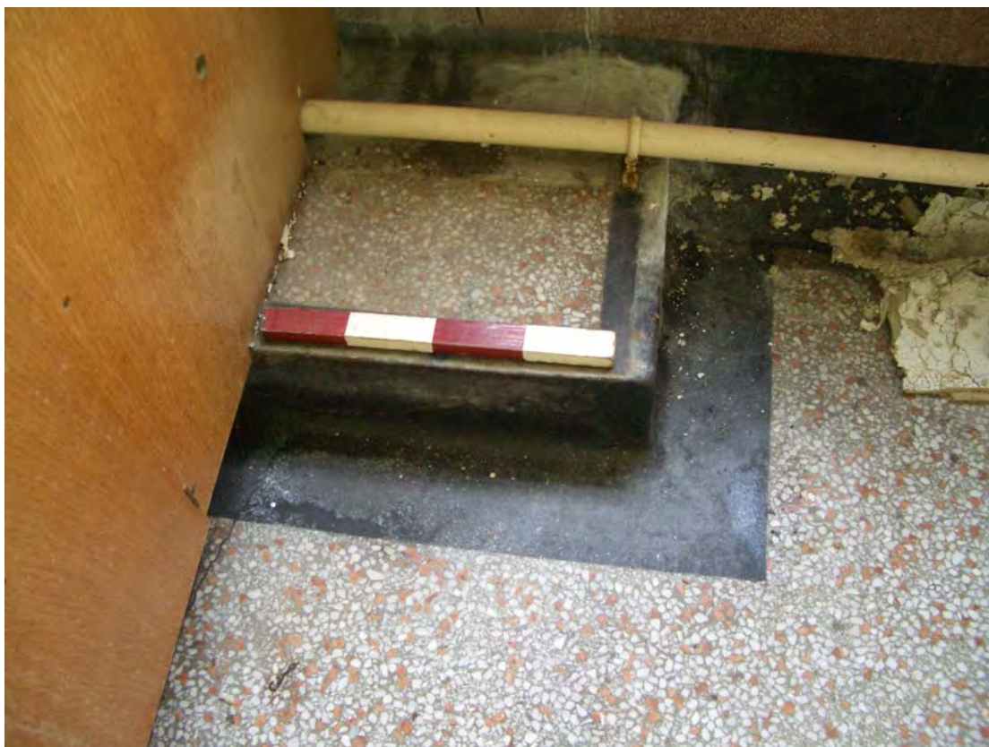
Plate 87. Head Office. First Floor Interior. Facing North.
