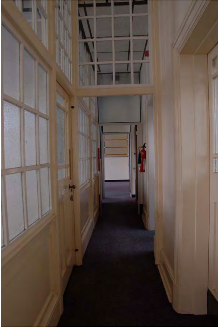
Plate 109. Head Office. First Floor Interior. Facing North.
