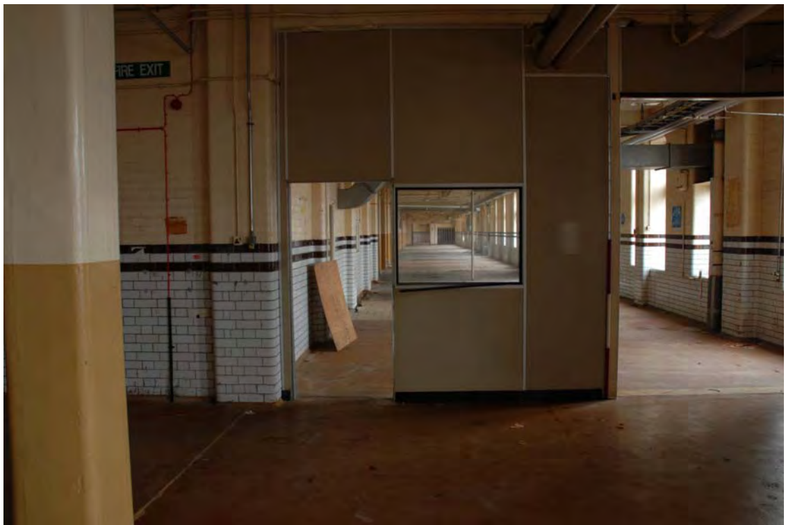
Plate 174. Factory. Third Floor Interior. Facing West.
