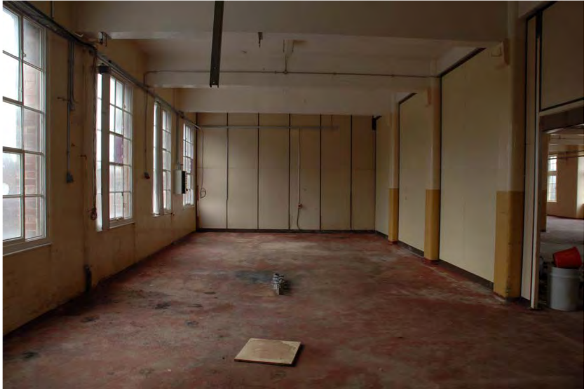
Plate 155. Factory. First Floor. Interior. Facing West.
