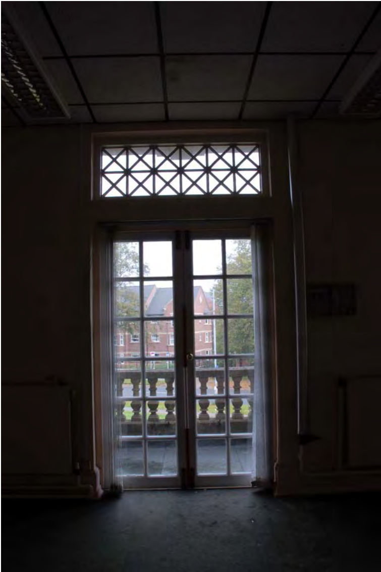
Plate 97. Head Office. First Floor Interior. Facing East.
