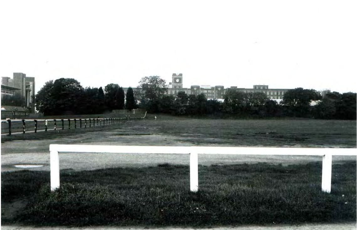
Plate 10. General View of Multi-Storey Factory. Facing North.
