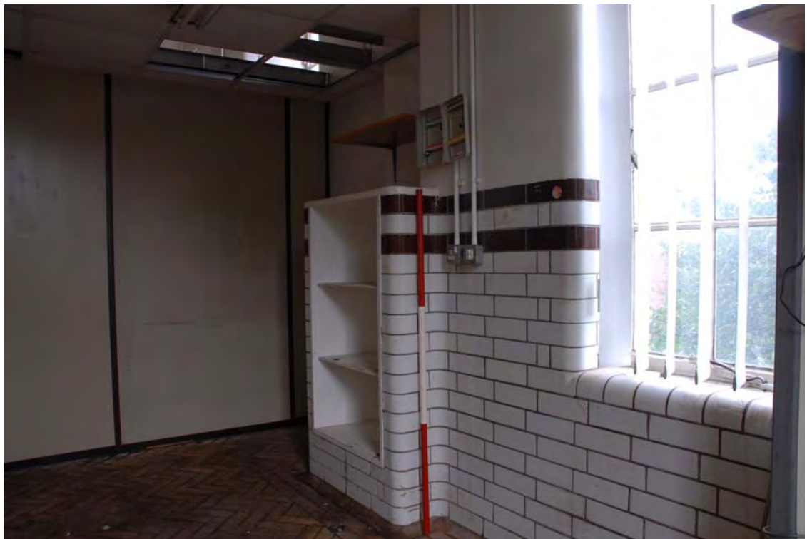
Plate 154. Factory. First Floor Interior. Facing South.
