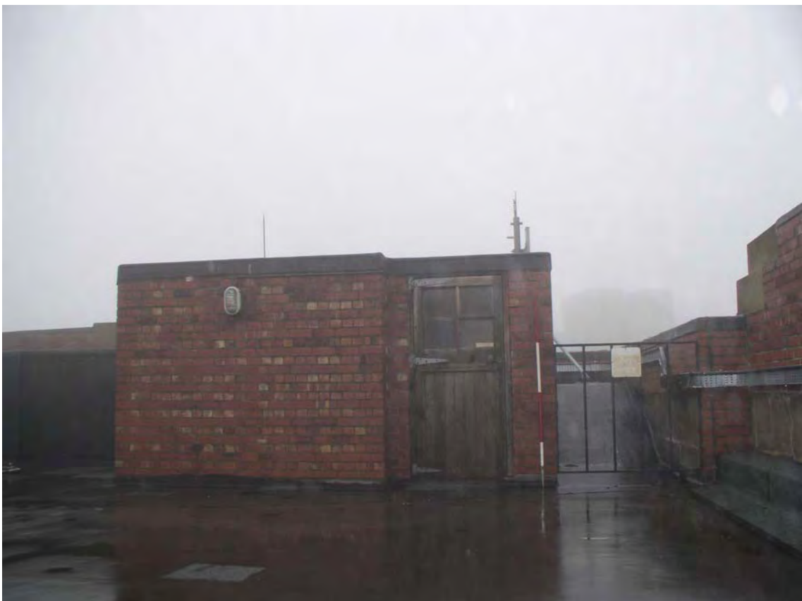
Plate 182. Factory. Roof. Facing West.
