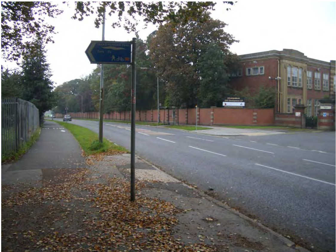
Plate 2. General View of Boundary Wall. Facing South-west.
