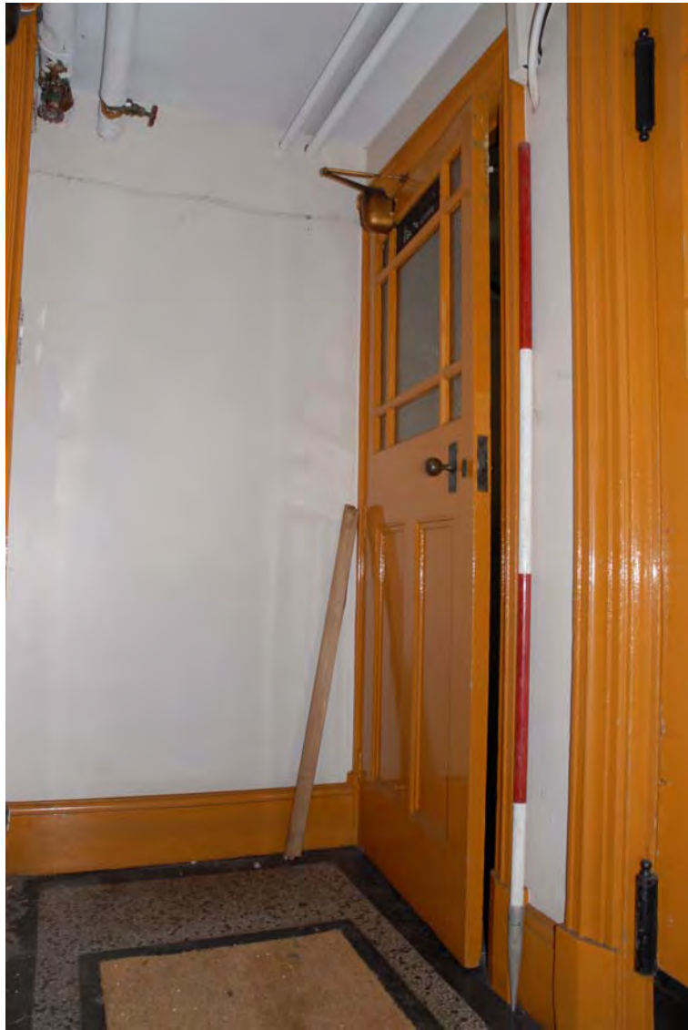
Plate 189. Head Office. Ground Floor. Basement Entrance. Facing North.
