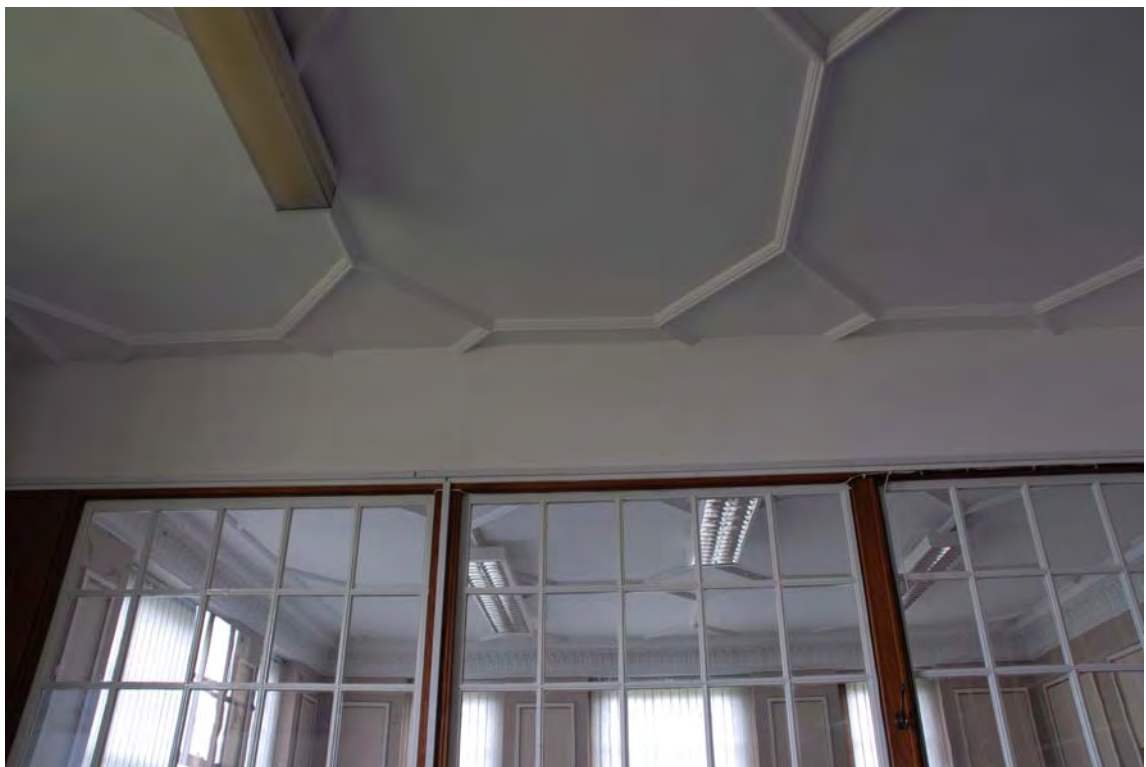
Plate 90. Head Office. First Floor Interior Ceiling. Facing East.
