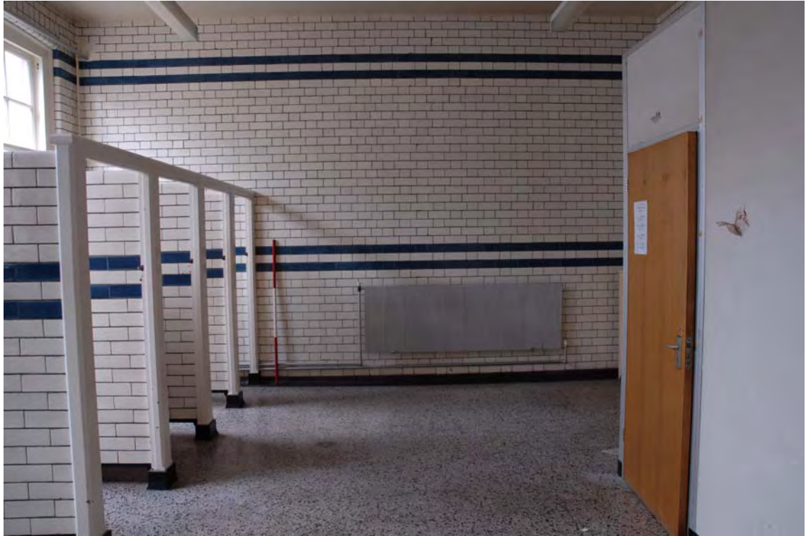
Plate 63. Head Office. First Floor Interior. Facing North.
