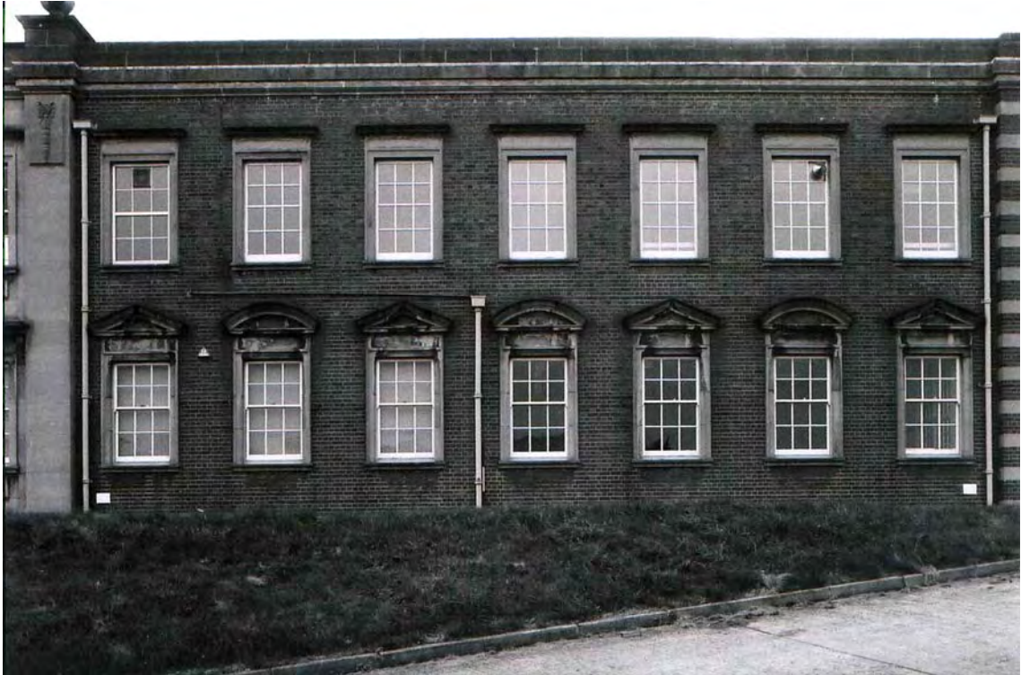
Plate 27. Head Office. South Elevation Windows. .Facing South.
