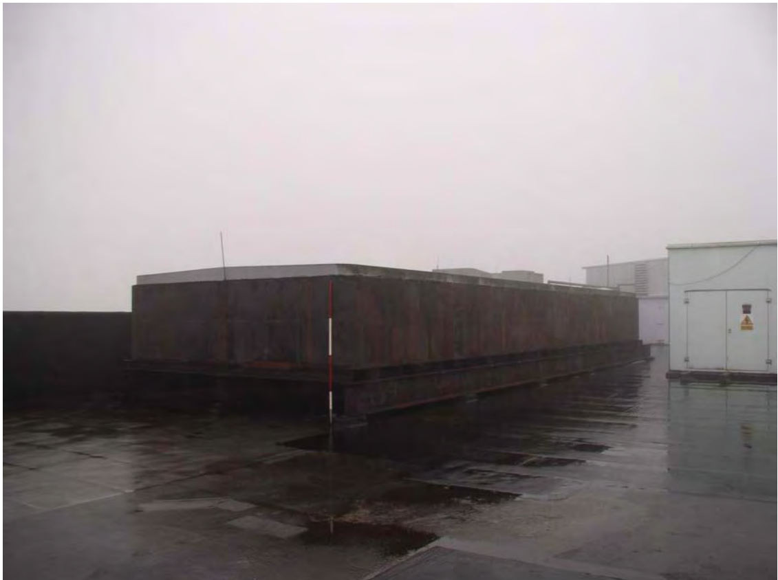
Plate 186. Factory. Roof. Facing South-west.
