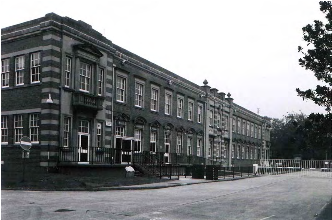
Plate 17. Head Office. South Elevation. Facing North-east.
