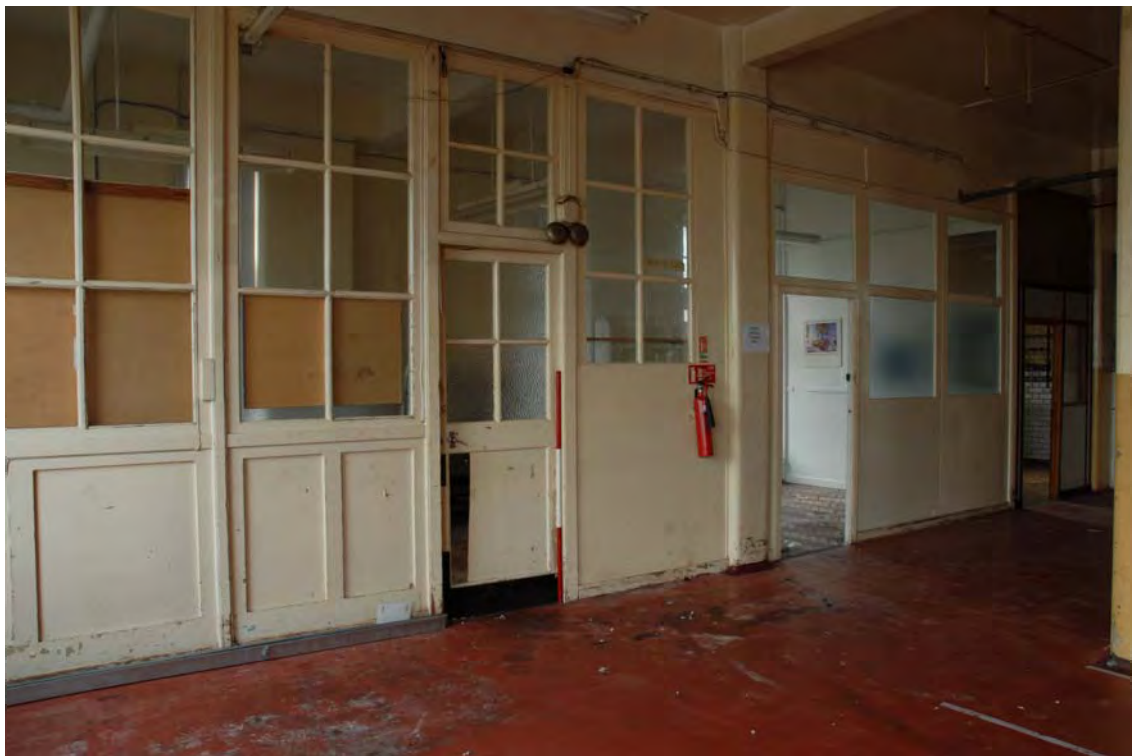
Plate 162. Factory. First Floor Interior. Facing West..
