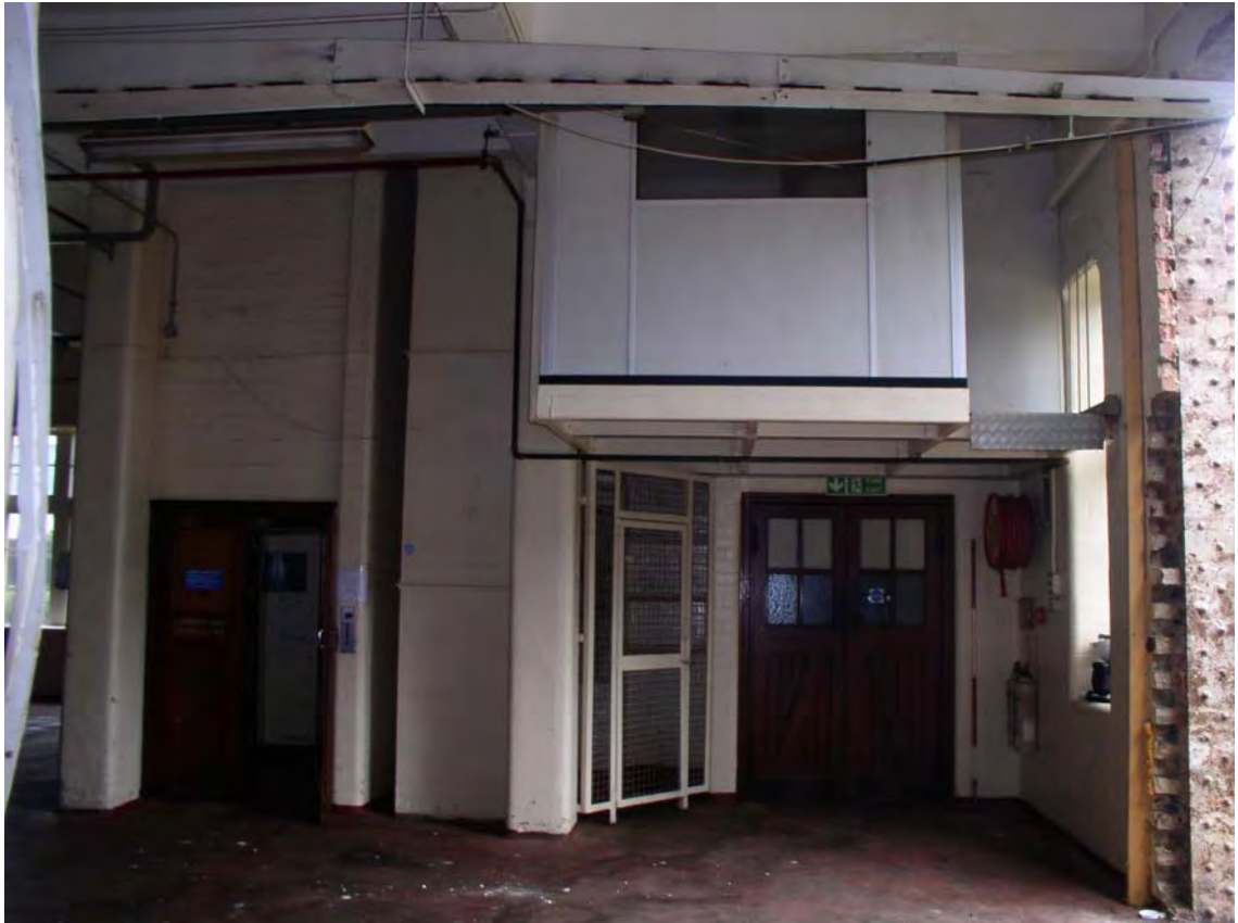
Plate 139. Factory. Ground Floor Interior. Facing North.
