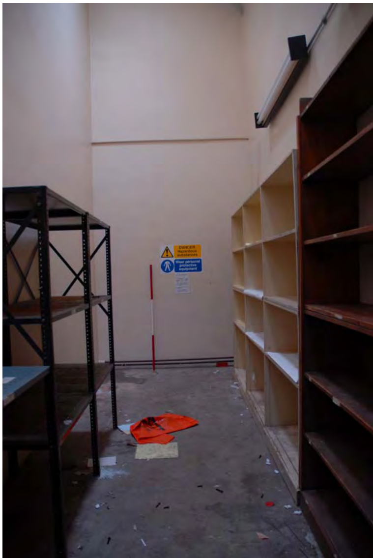
Plate 115. Head Office. First Floor Interior. Facing East.
