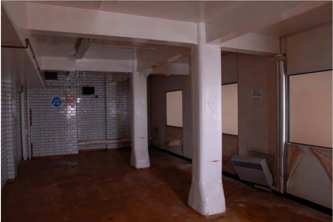
Plate 159. Factory. First Floor Interior. Facing North.
