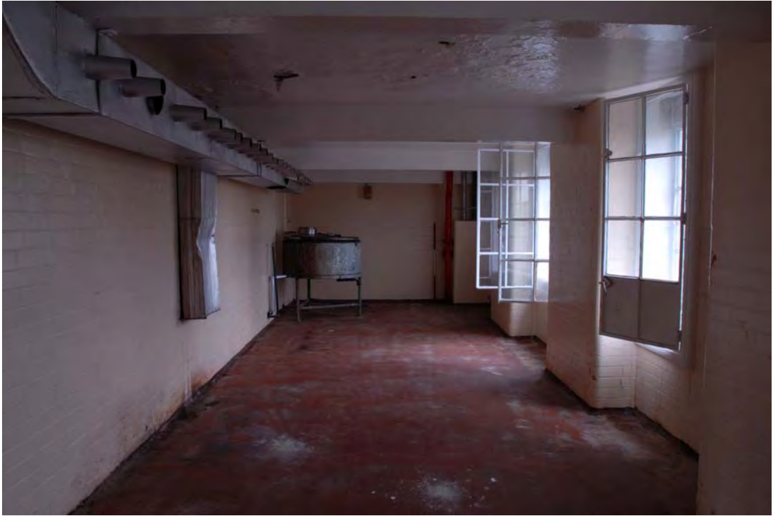
Plate 167. Factory. Second Floor Interior. Facing West.
