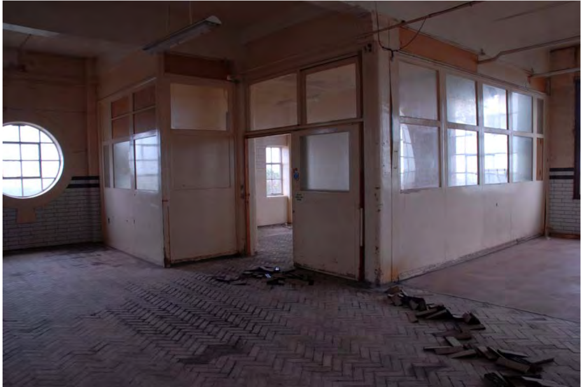
Plate 181. Factory. Fourth Floor Interior. Facing South-east.
