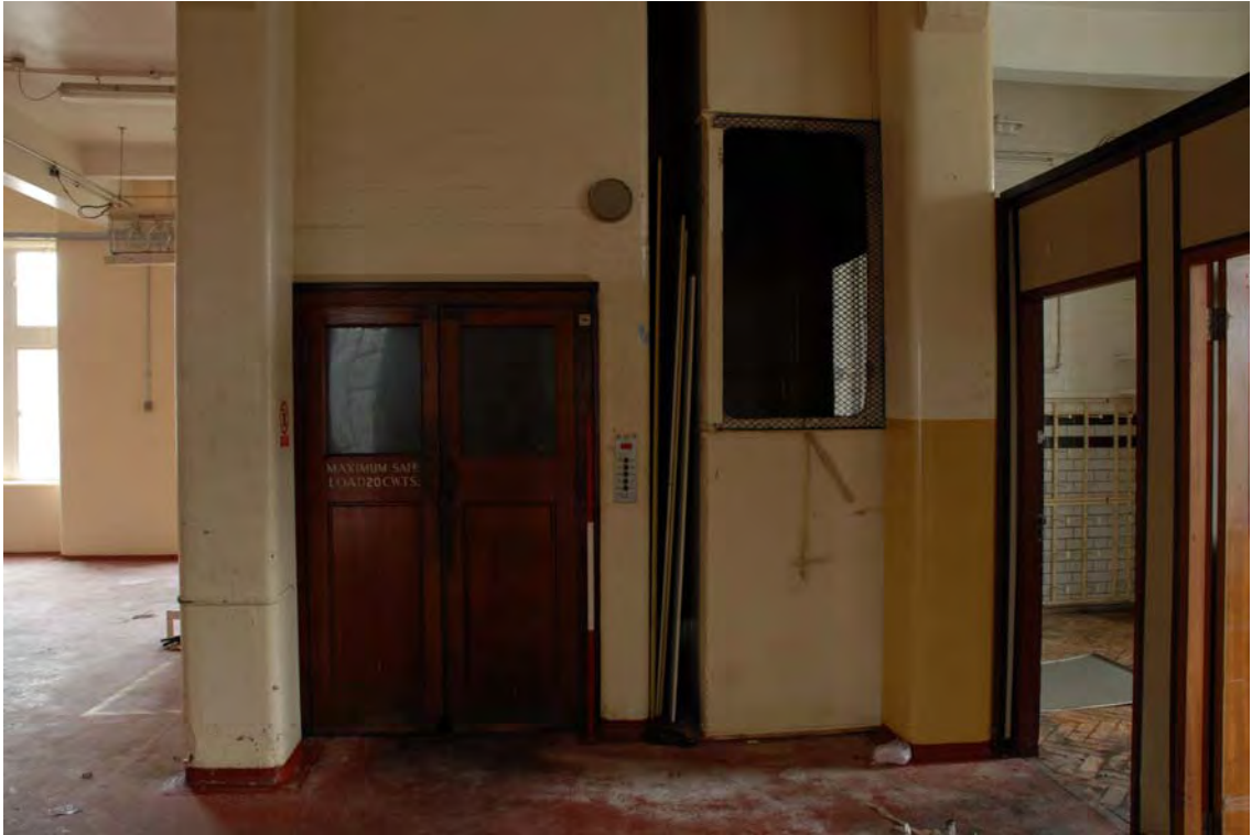
Plate 153. Factory. First Floor Interior. Facing North.
