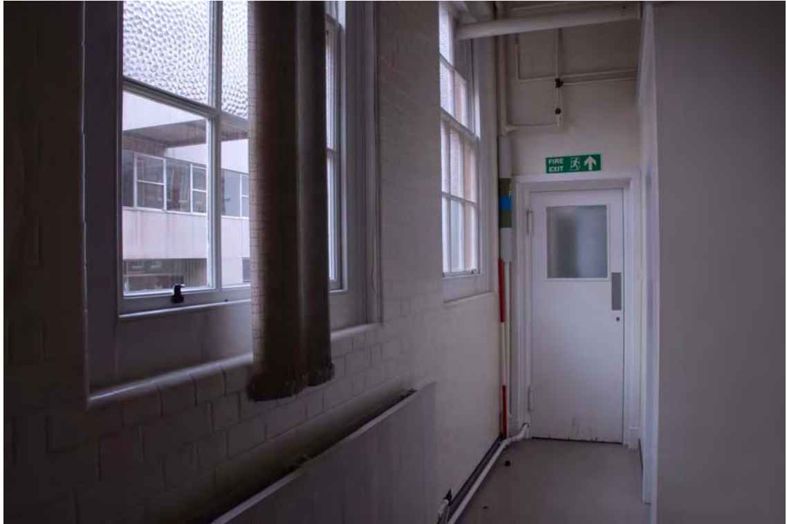
Plate 57. Head Office. Ground Floor Interior. Facing North.
