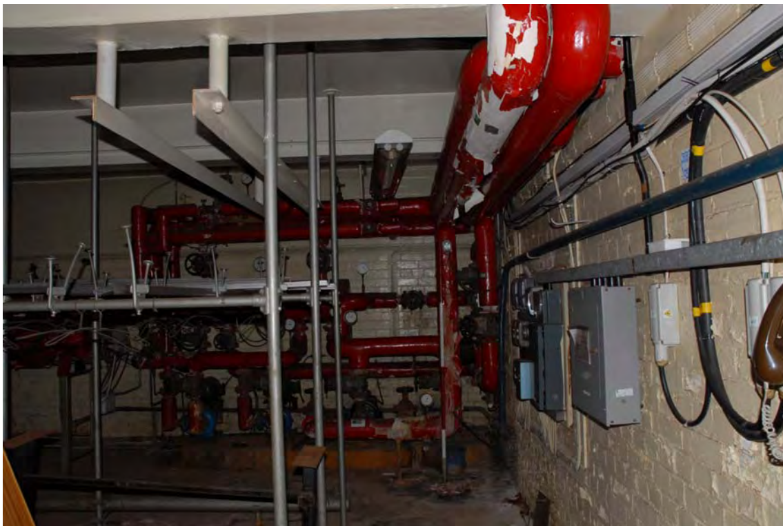
Plate 190. Head Office. Basement. Facing North.
