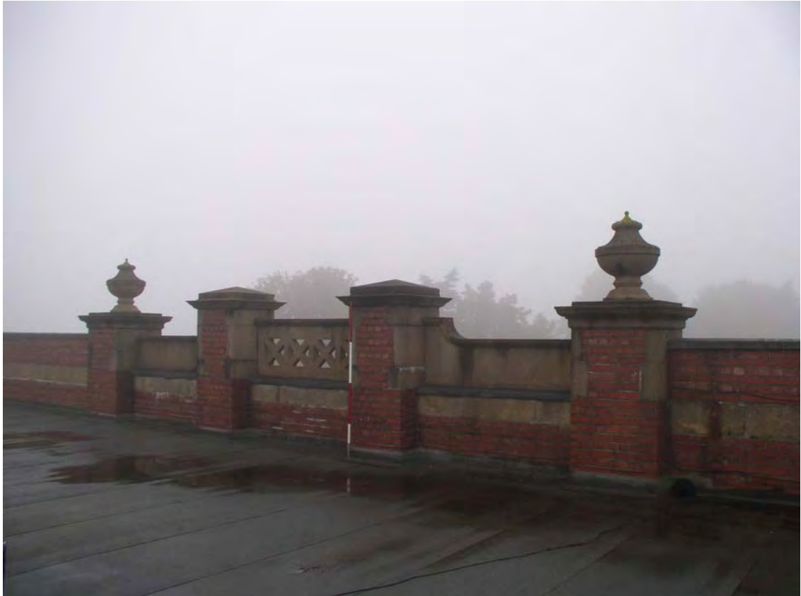
Plate 121. Head Office Roof. Facing South.
