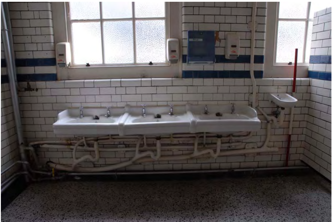
Plate 68. Head Office. First Floor Interior. Facing West.
