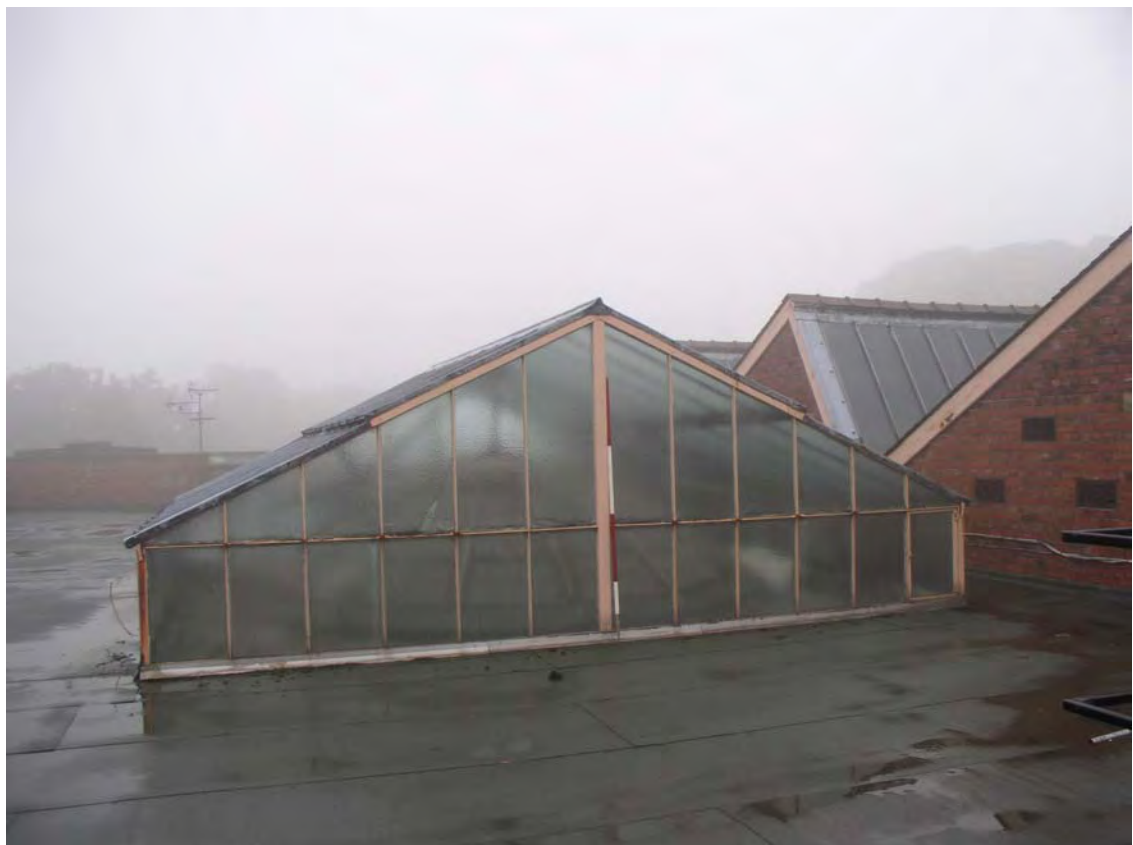
Plate 122. Head Office Roof. Facing North.
