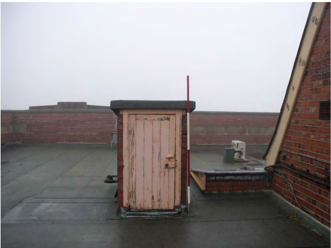
Plate 120. Head Office Roof. Facing North.
