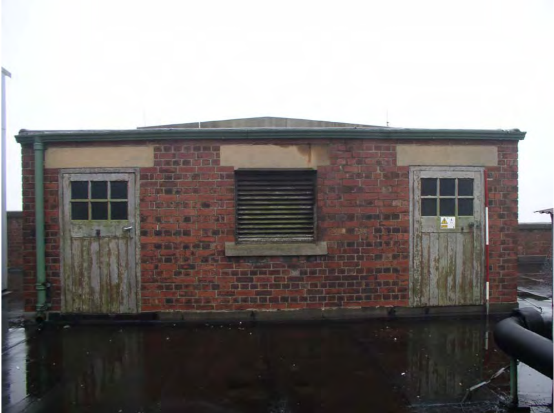
Plate 185. Factory. Roof. Facing South.
