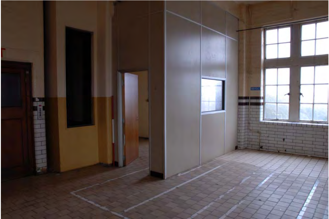
Plate 173. Factory. Third Floor Interior. Facing North-east.
