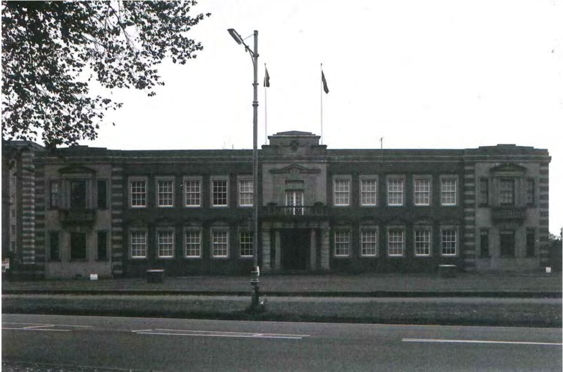
Plate 11. Head Office. East Elevation. Facing West.
