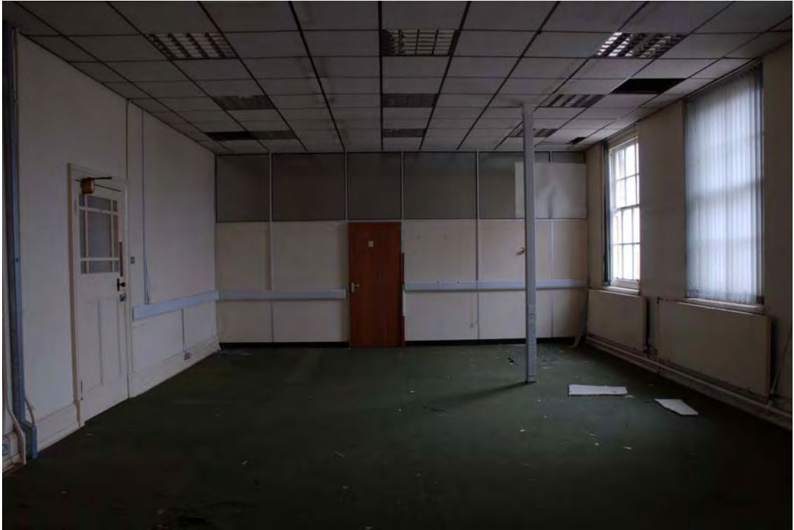
Plate 107. Head Office. First Floor Interior. Facing East.
