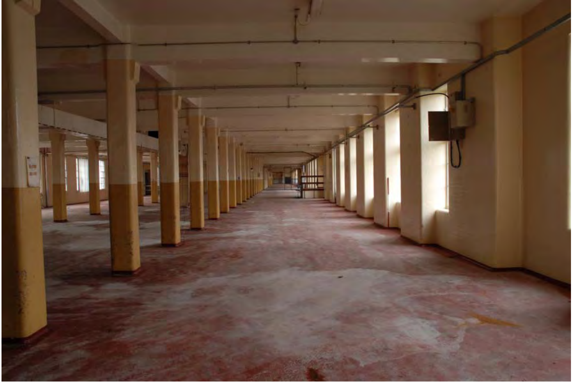
Plate 151. Factory. First Floor Interior. Facing West.
