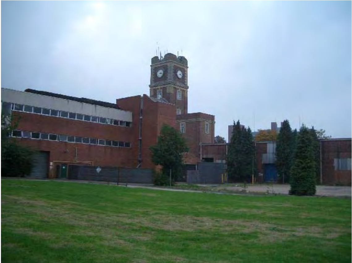
Plate 9. General View of Clock Tower. Facing South-west.
