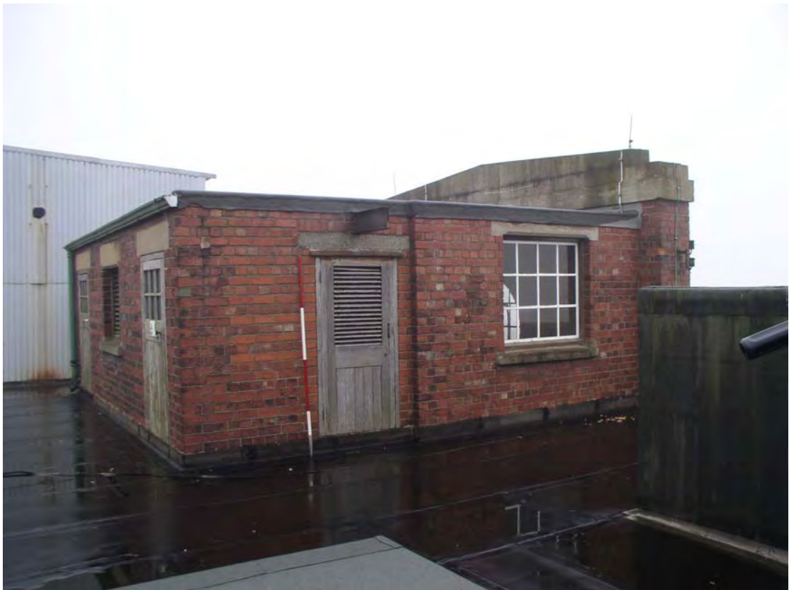
Plate 184. Factory. Roof. Facing East.
