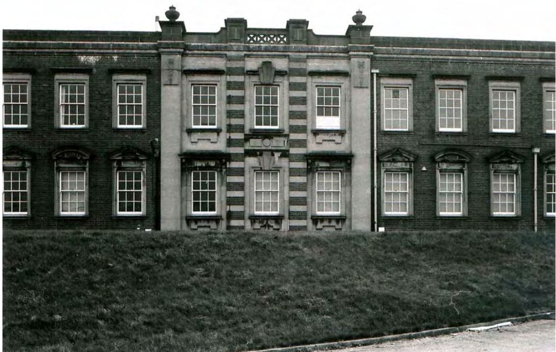
Plate 24. Head Office. South Elevation Centre. Facing South.
