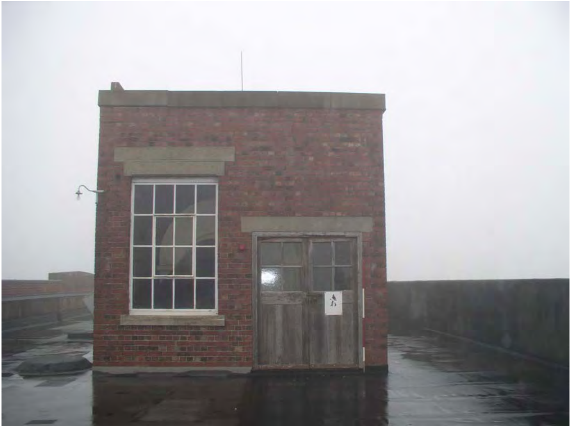
Plate 183. Factory. Roof. Facing East.
