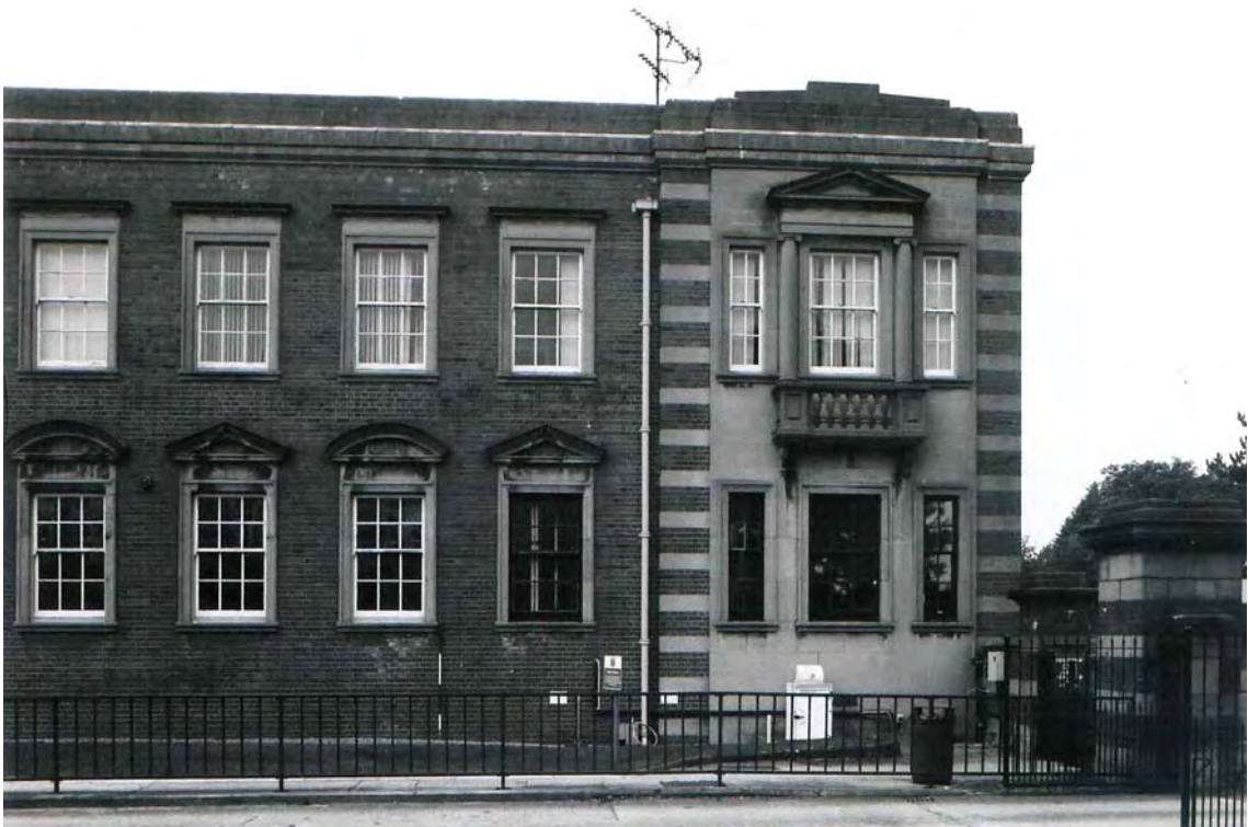
Plate 20. Head Office. South Elevation East End. Facing North.
