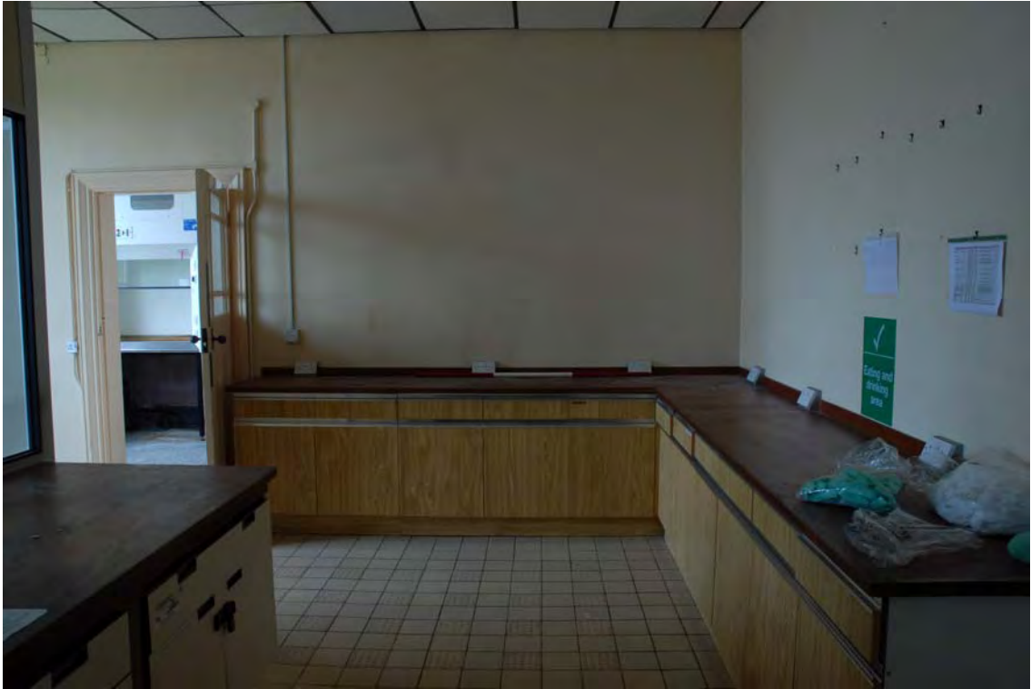
Plate 81. Head Office. First Floor. Interior. Facing East.
