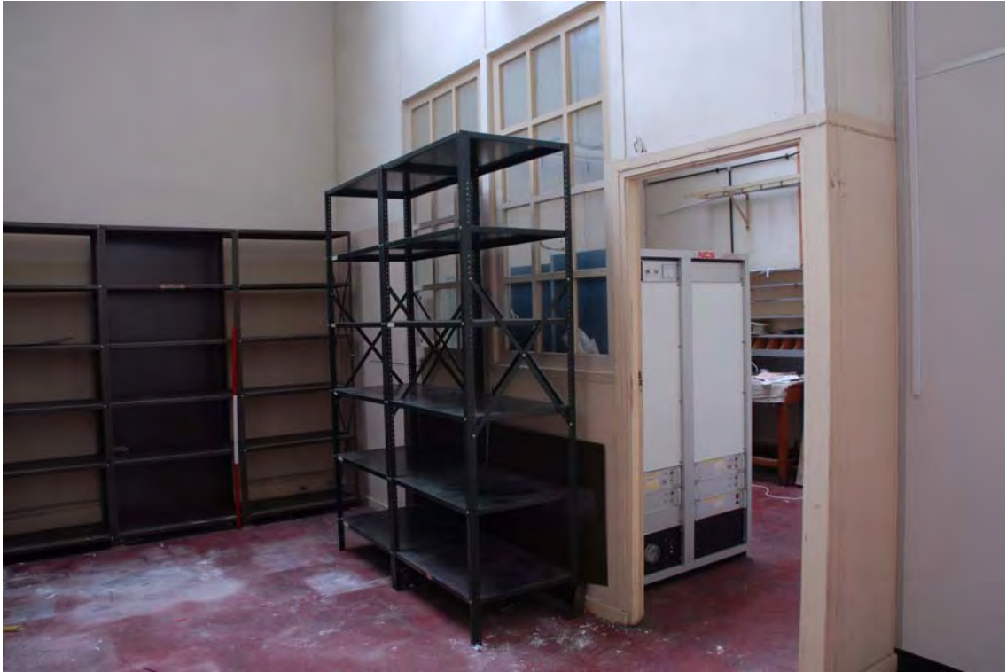
Plate 113. Head Office. First Floor Interior. Facing North-east.
