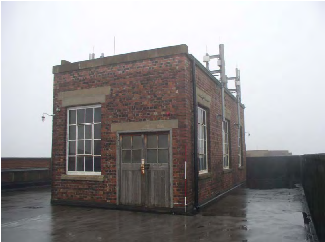
Plate 187. Factory. Roof. Facing East.
