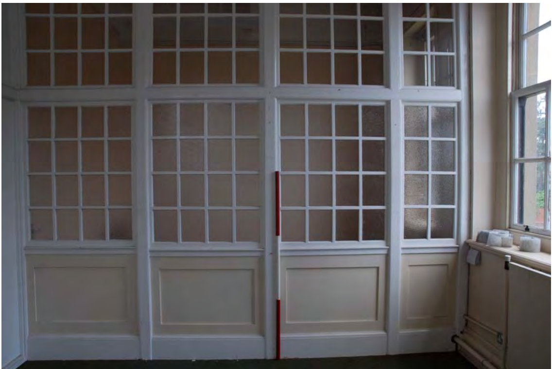
Plate 102. Head Office. First Floor Interior. Facing North.
