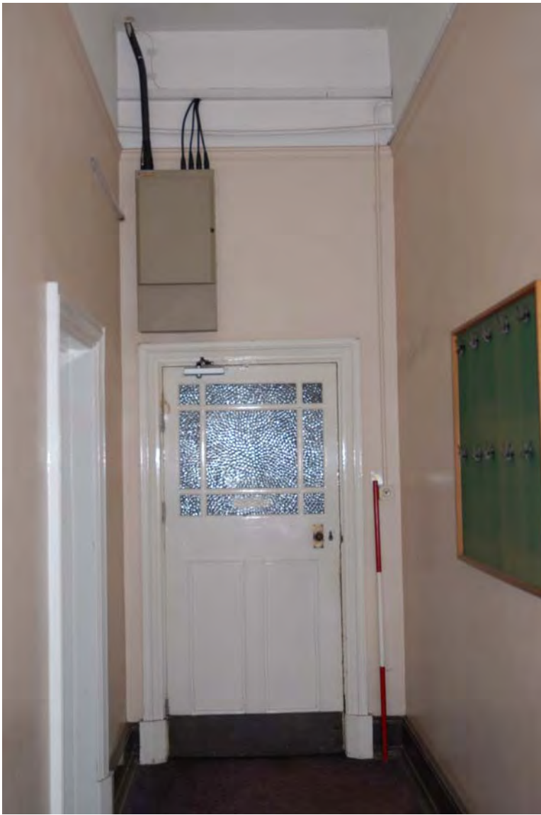
Plate 51. Head Office. Ground Floor Interior. Facing North.
