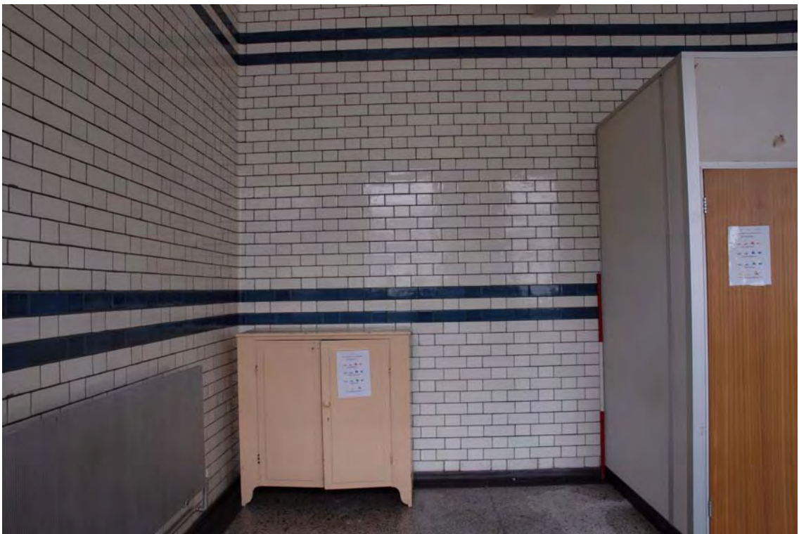
Plate 66. Head Office. First Floor Interior. Facing East.
