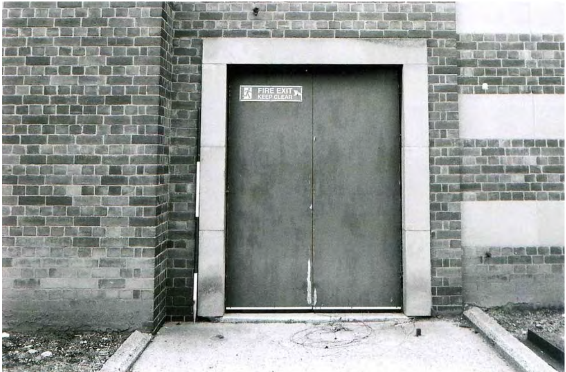
Plate 132. Factory. East Elevation. Facing West.
