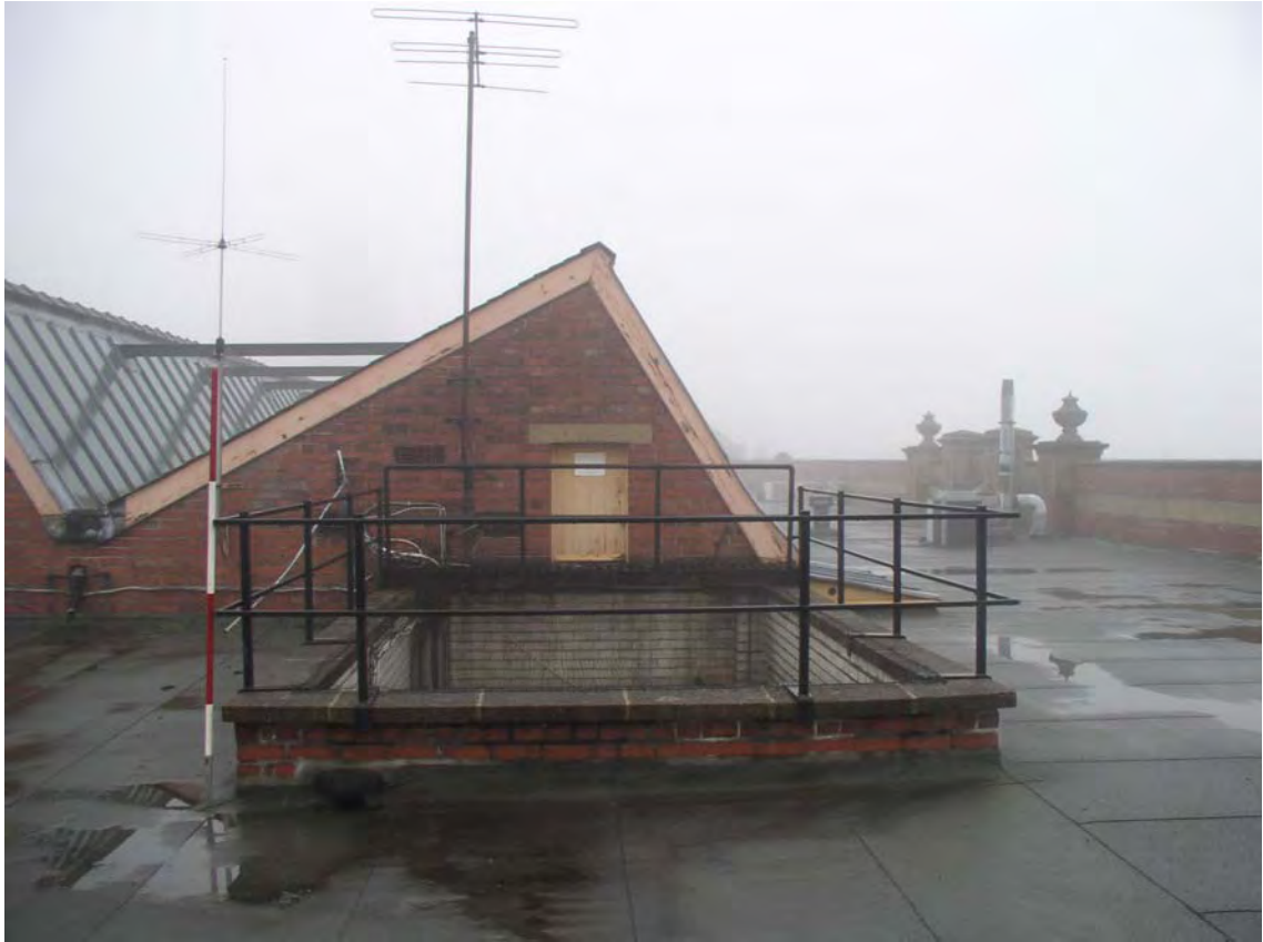
Plate 123. Head Office Roof. Facing West.
