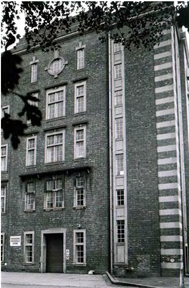
Plate 128. Factory. North Elevation. Facing South.
