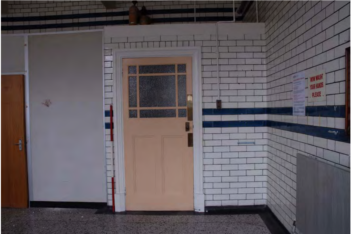
Plate 67. Head Office. First Floor Interior. Facing East.
