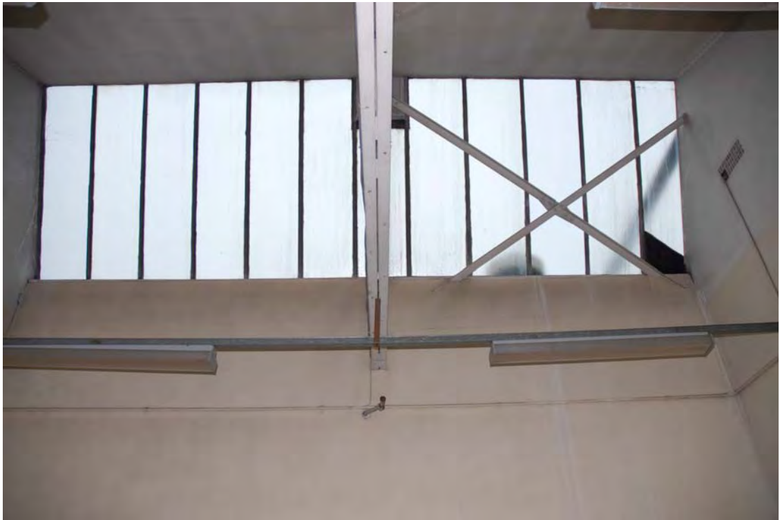
Plate 112. Head Office. First Floor Interior. Facing North.
