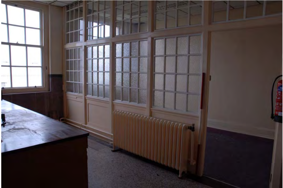
Plate 85. Head Office. First Floor Interior. Facing North-east.
