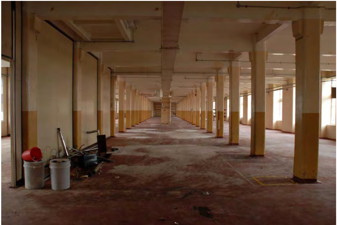
Plate 152. Factory. First Floor Interior. Facing West.
