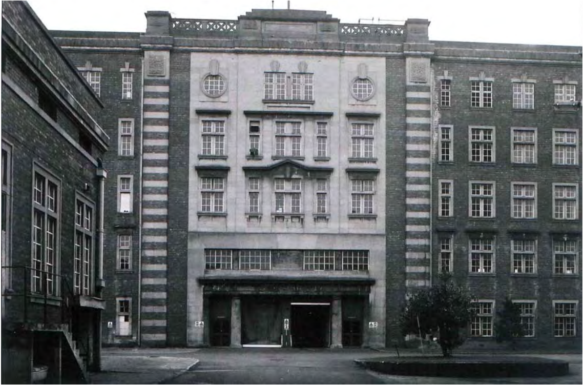
Plate 127. Factory. North Elevation. Facing South.
