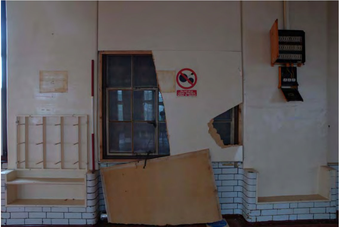
Plate 161. Factory. First Floor Interior. Facing North.
