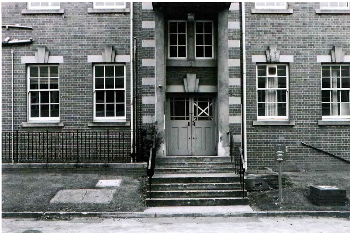
Plate 30. Head Office. West Elevation Door. Facing East.
