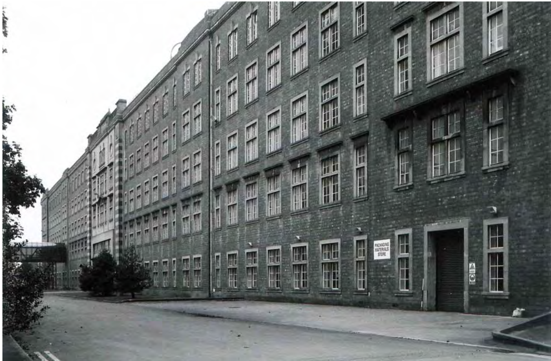
Plate 126. Factory. North Elevation. Facing East.
