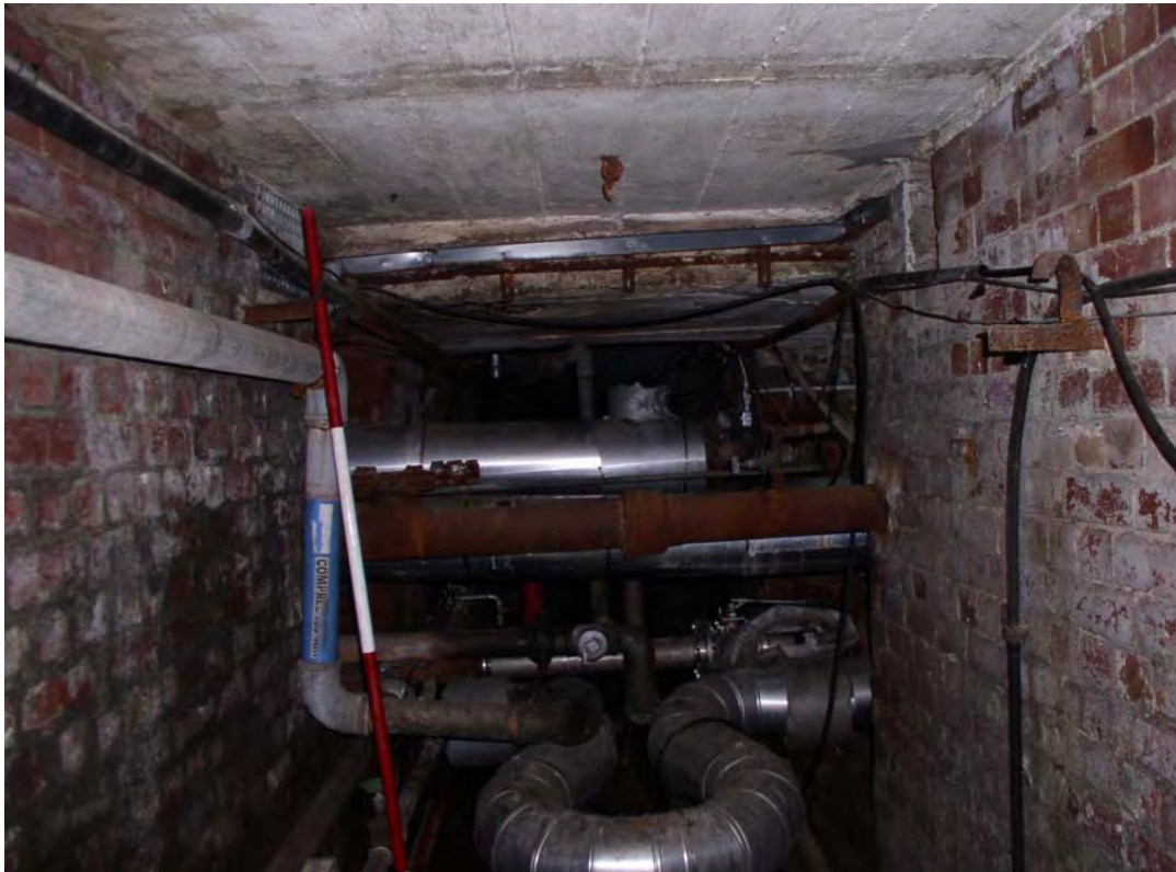
Plate 136. Factory. Basement. Facing East.
