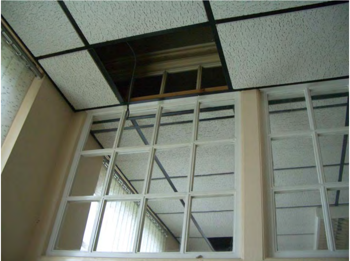
Plate 93. Head Office. First Floor Interior. Facing East.
