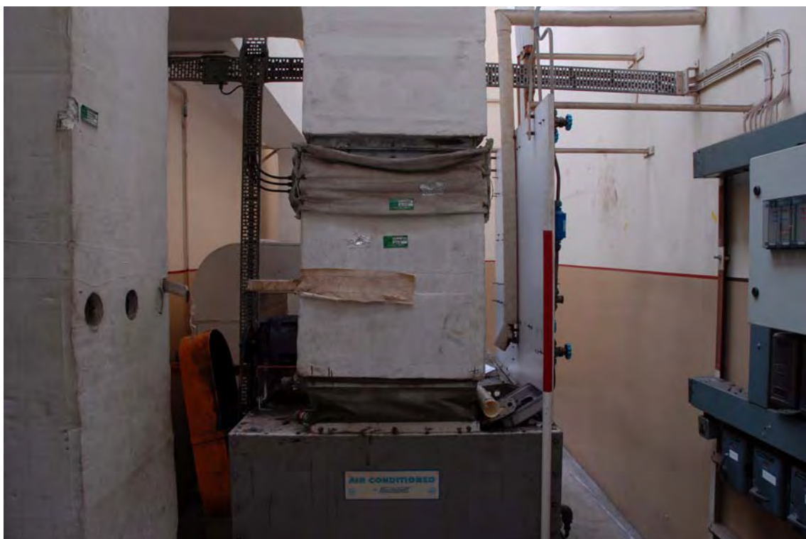
Plate 116. Head Office. First Floor Interior. Facing East.
