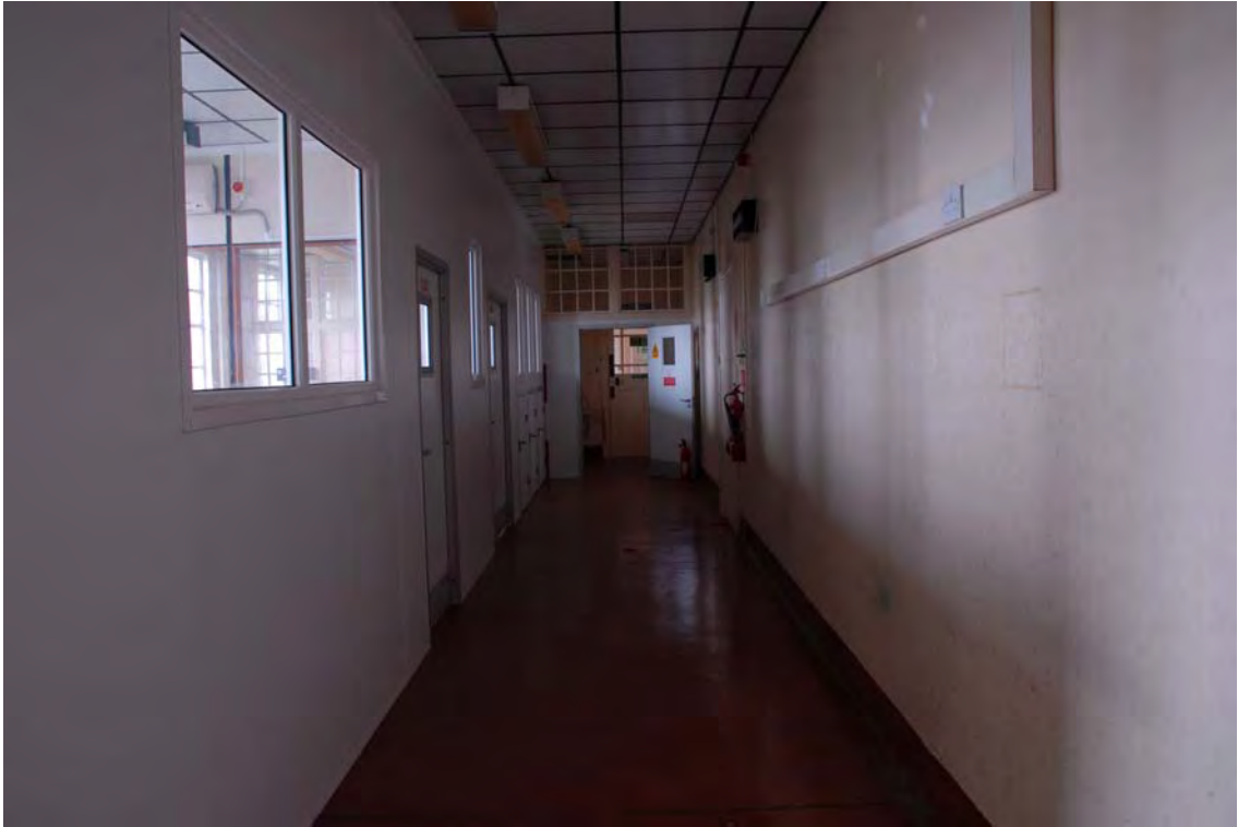
Plate 79. Head Office. First Floor Interior. Facing East.
