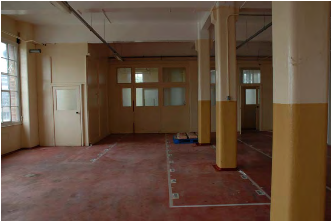
Plate 168. Factory. Second Floor Interior. Facing West.
