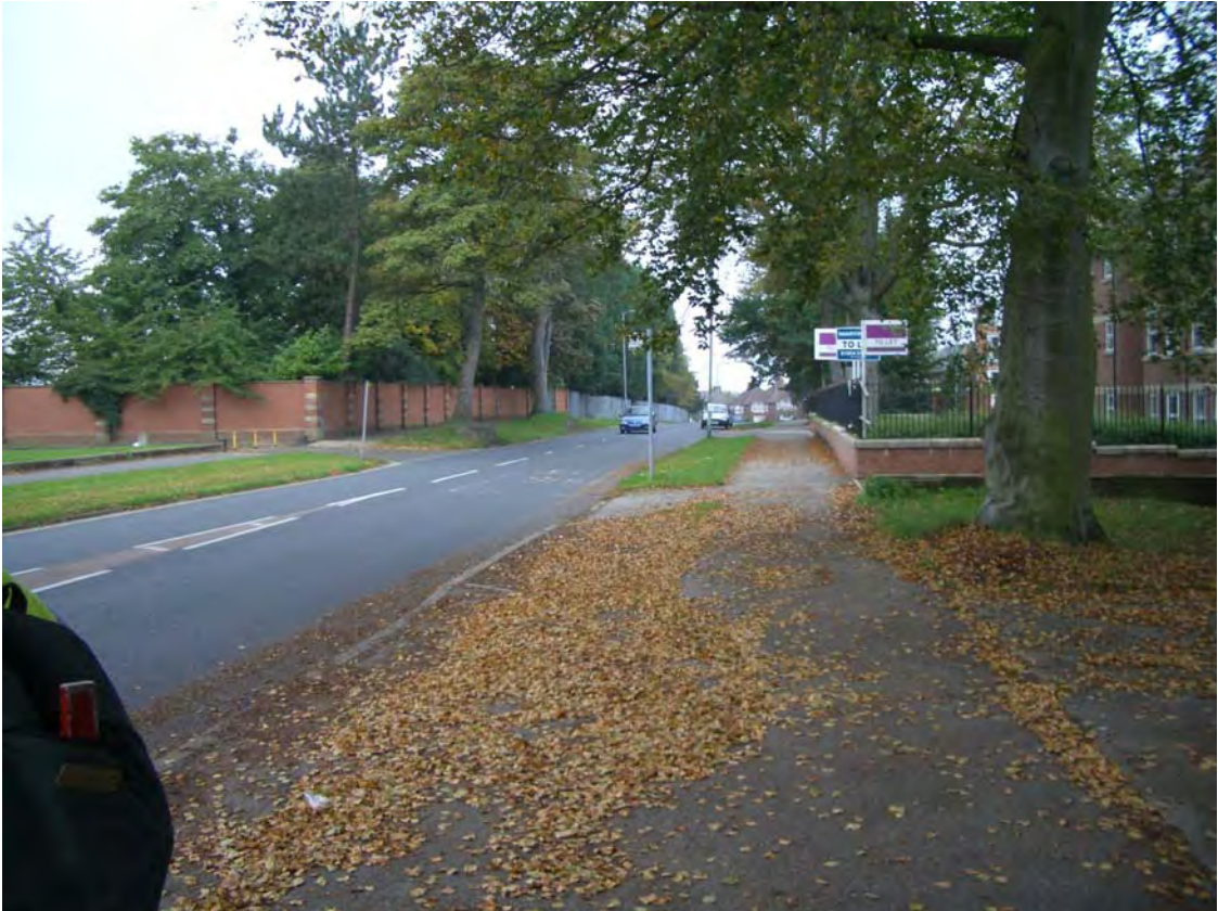
Plate 3. General View of Boundary Wall. Facing North-west.
