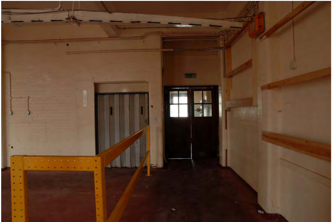
Plate 158. Factory. First Floor Interior. Facing South.
