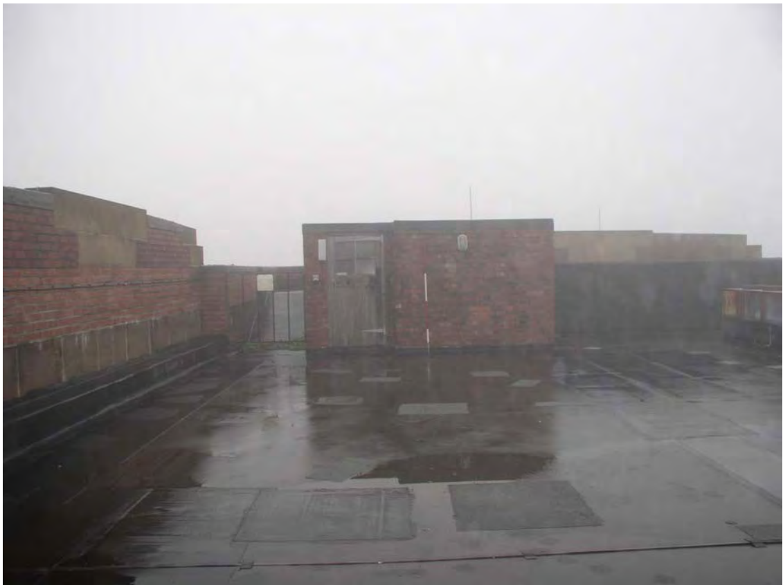
Plate 188. Factory. Roof. Facing East.
