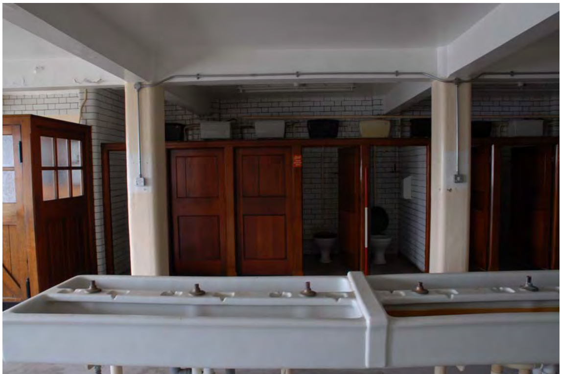
Plate 170. Factory. Second Floor Interior. Facing West.
