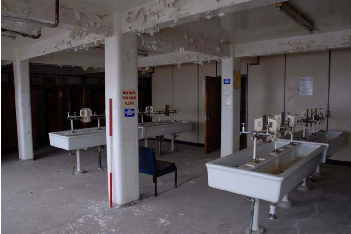
Plate 175. Factory. Third Floor Interior. Facing West.
