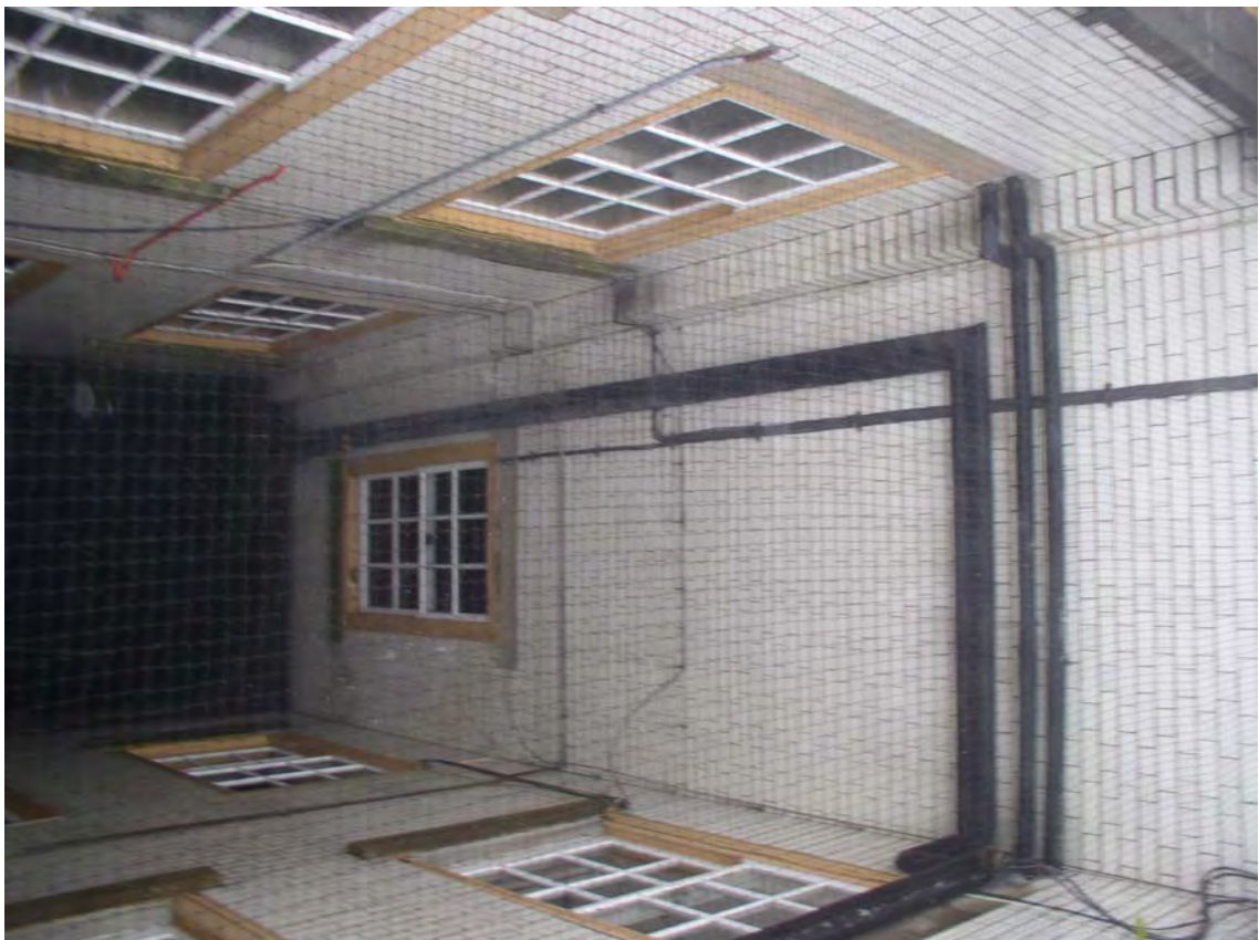
Plate 124. Head Office Roof. Facing West.
