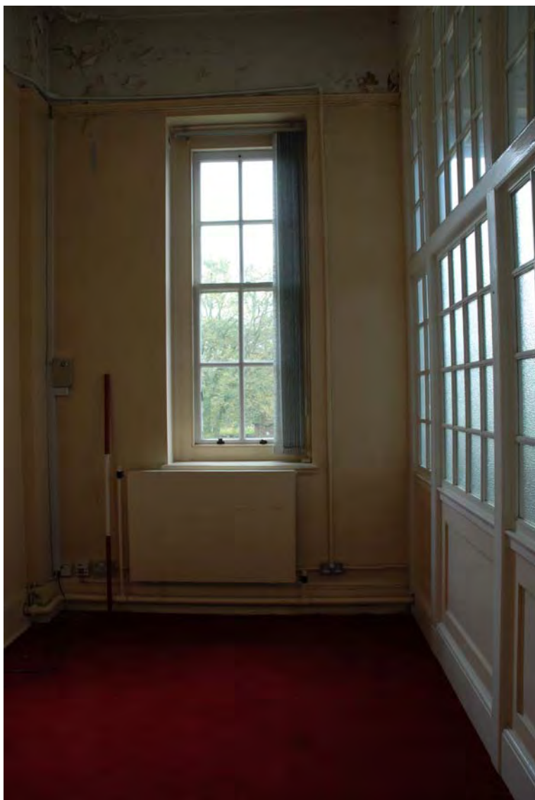
Plate 103. Head Office. First Floor Interior. Facing North.
