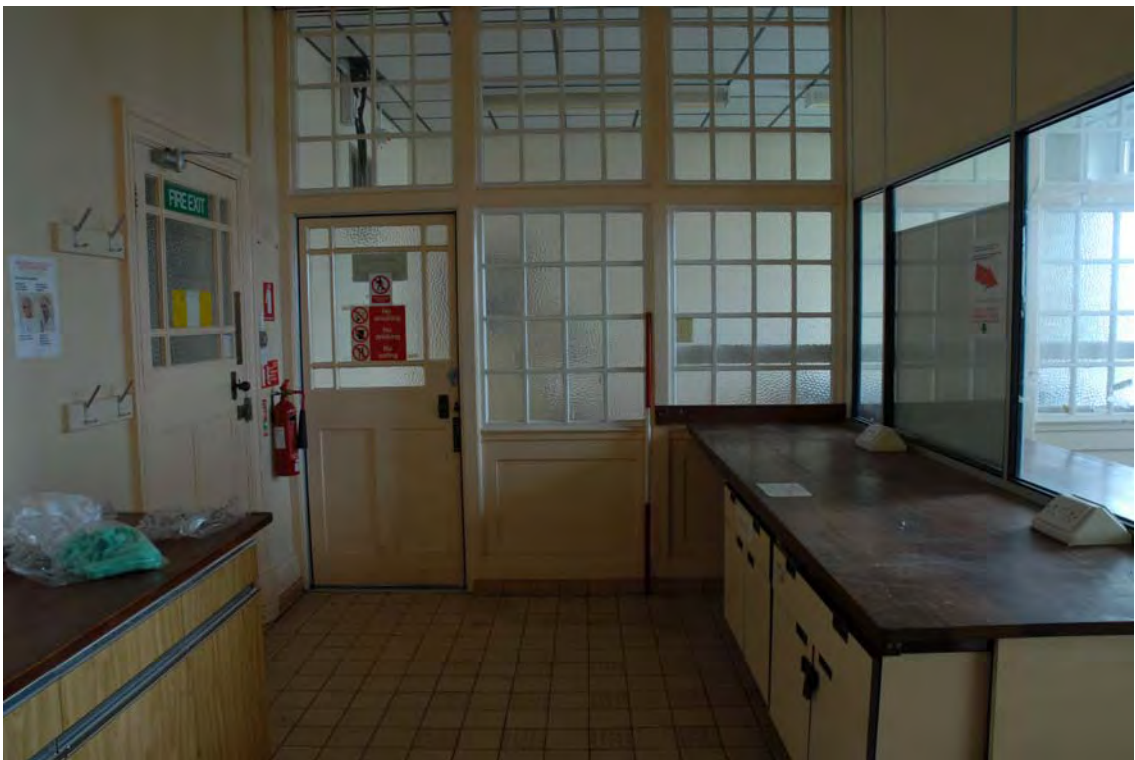
Plate 82. Head Office. First Floor. Interior. Facing West.
