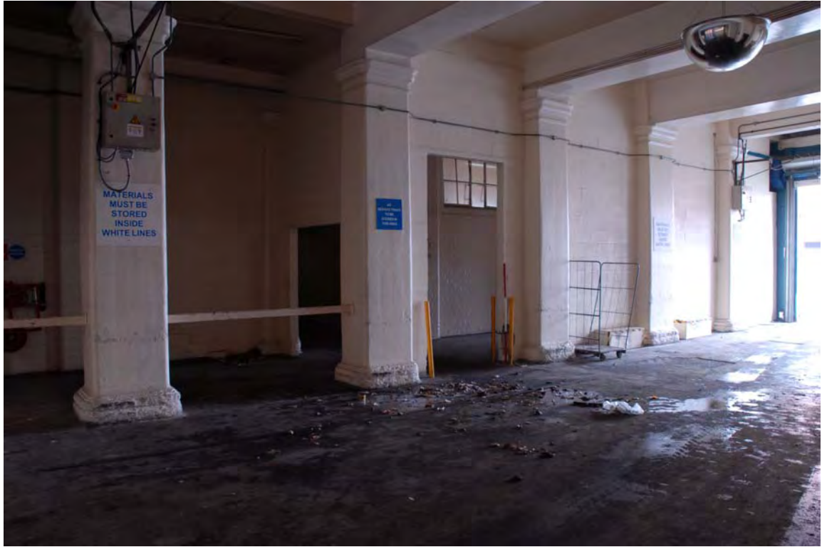
Plate 145. Factory. Ground Floor Interior. Facing North-east.
