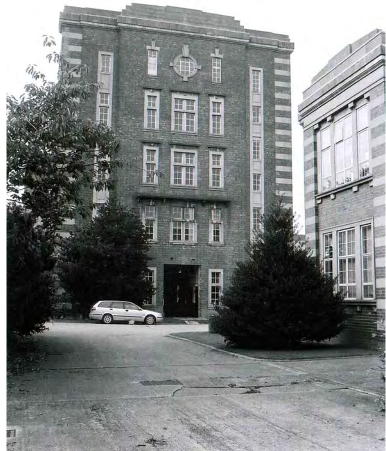
Plate 130. Factory. East Elevation. Facing West.
