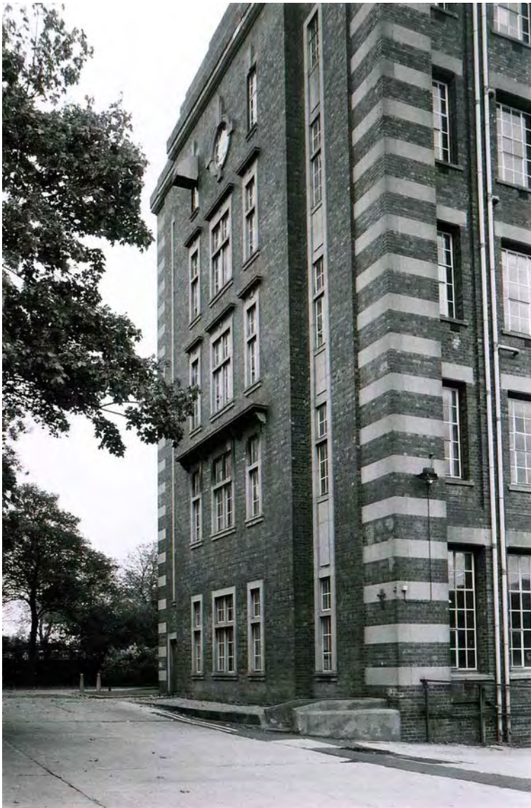
Plate 133. Factory. West Elevation. Facing South-east.
