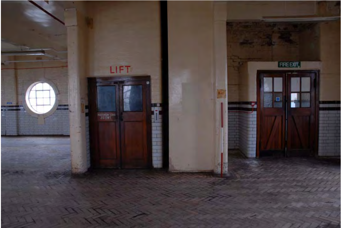
Plate 179. Factory. Fourth Floor Interior. Facing North.
