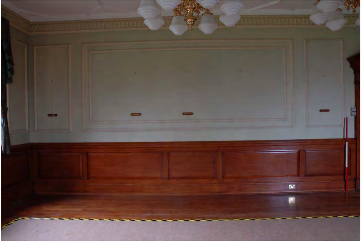
Plate 43. Head Office. Ground Floor Interior. Facing South.
