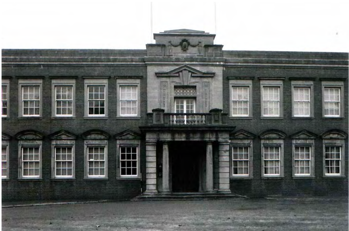
Plate 12. Head Office. East Elevation. Centre. Facing West.
