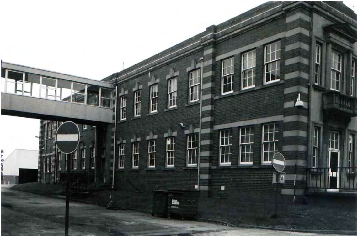
Plate 29. Head Office. West Elevation. Facing North-east.
