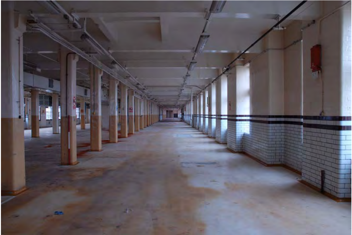
Plate 163. Factory. Second Floor Interior. Facing West.
