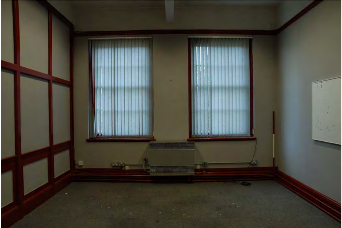
Plate 101. Head Office. First Floor Interior. Facing East.
