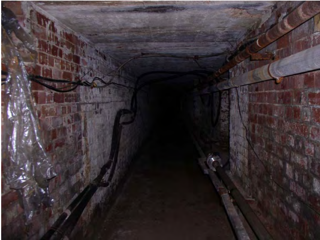
Plate 137. Factory. Basement. Facing West.
